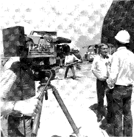
Left spillway media inspection, Glen Canyon Dam.
