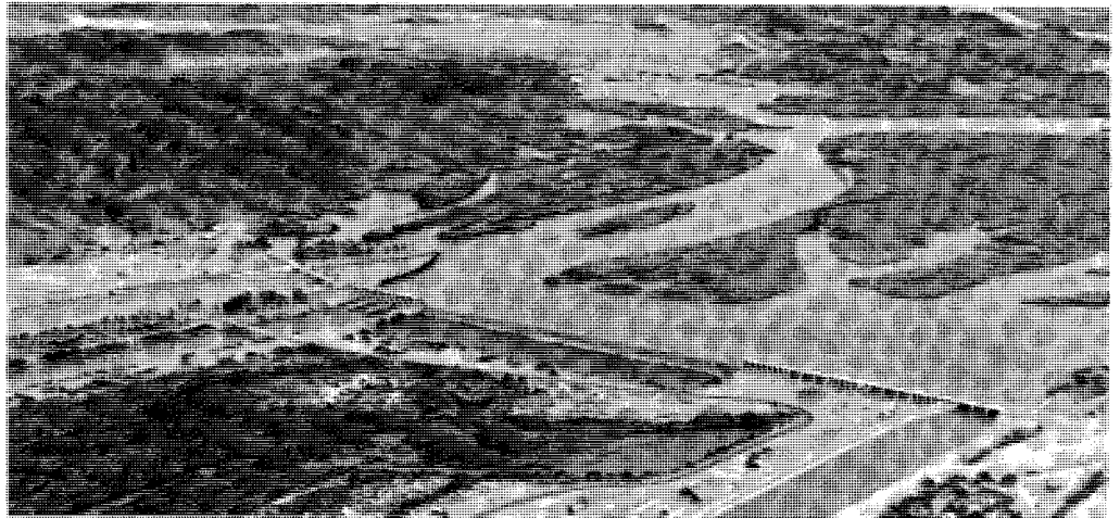
Imperial Dam with Senator Wash Dam in upper background, California.
