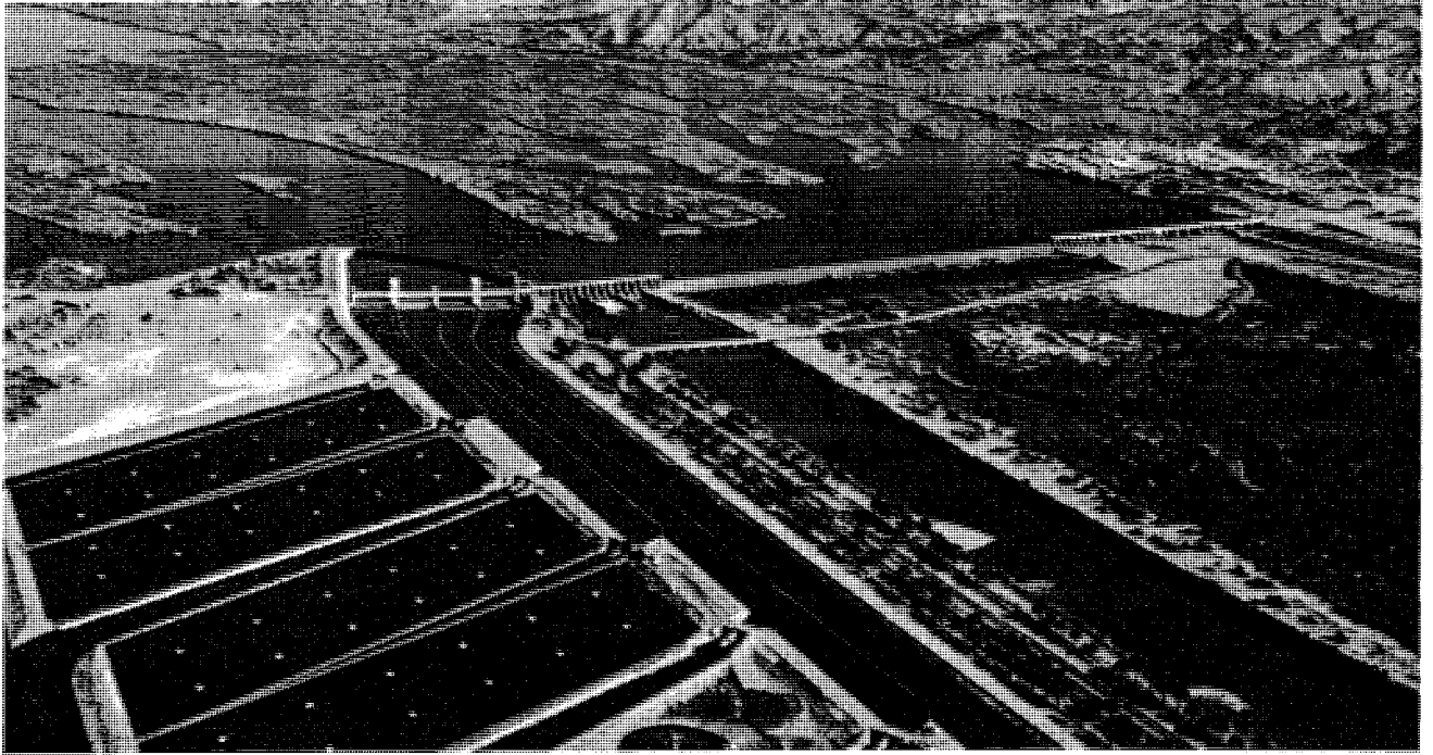
Imperial Dam and desilting works, Arizona-California
