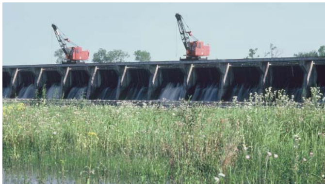
Wildflowers enliven the lakeside of the structure during spring high water.
