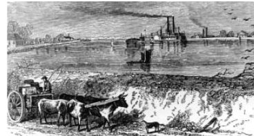
By the early 1800s, levees provided a measure of protection.
