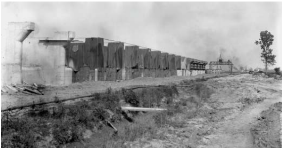
High strength concrete used in the spillway was an engineering advancement.
