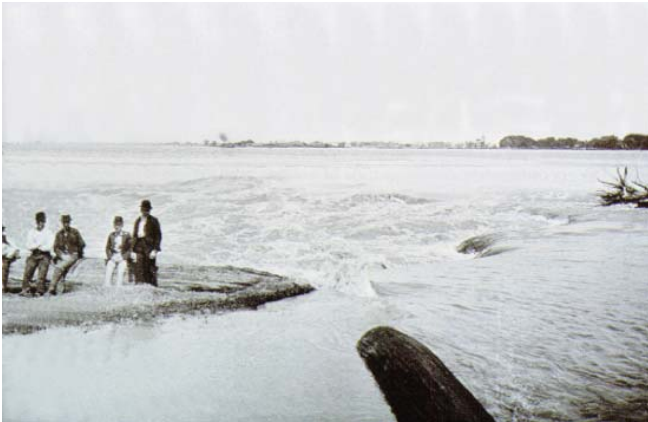
Breaking through the levee just above New Orleans, the river at Ames Crevasse in 1891 flooded much of western Jefferson Parish.
