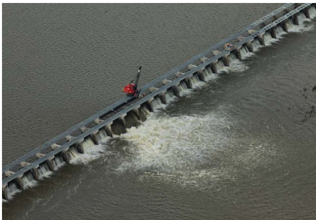
Map of Bonnet Carré Spillway (top), and aerial of the spillway in operation during the flood of 2011 (bottom).
