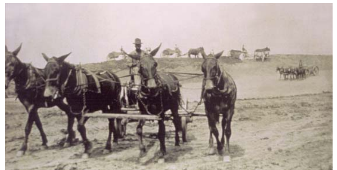
Early levee construction
