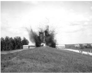
With MRC approval, Gov. Simpson gave the "go ahead" to dynamite the Caernarvon levee below New Orleans to create an artificial crevasse during the 1927 flood. The effort not only saved the city, it also blew away the "levees only" policy of the MRC.
