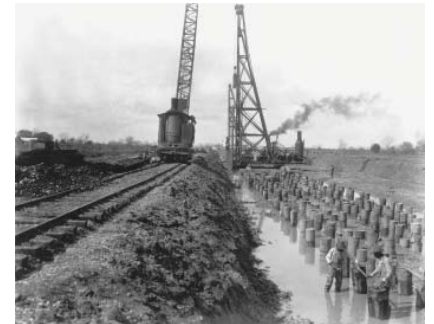
Thousands of wooden pilings were driven to provide a reliable foundation for the spillway structure.
