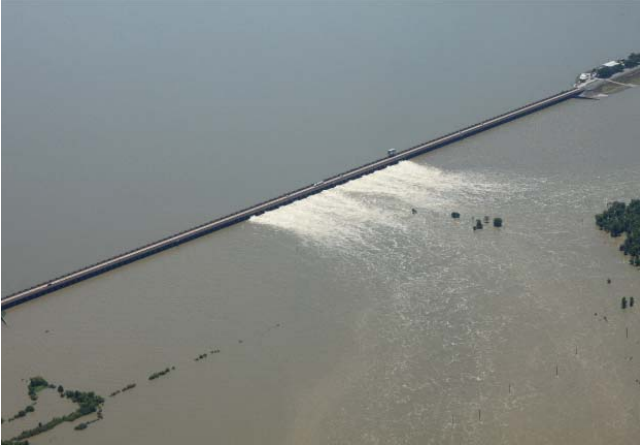
The Corps operated the Morganza Floodway for only the second time ever (and the first time for its intended purpose) in 2011 to divert excess Mississippi River water to the Atchafalaya River Basin and relieve pressure on the mainline Mississippi River levees.
