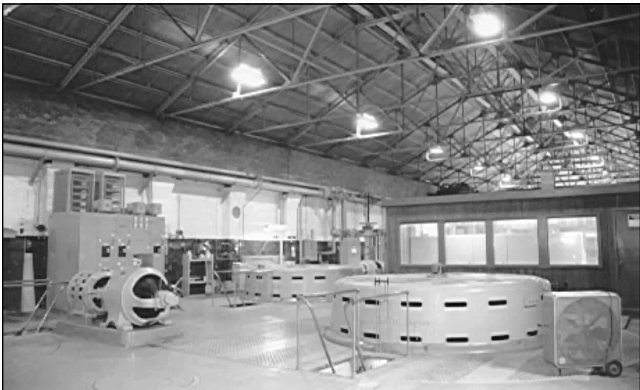
Figure 64. Drainage Pumping Station No. 7. View of interior, showing motor covers of 250 cfs centrifugal “flathead” pumps.
