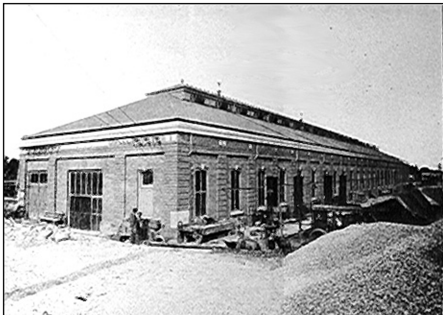
Figure 53. Drainage Pumping Station No. 6, after 1914 and 1929 extensions (from Sewerage & Water Board 1929).
