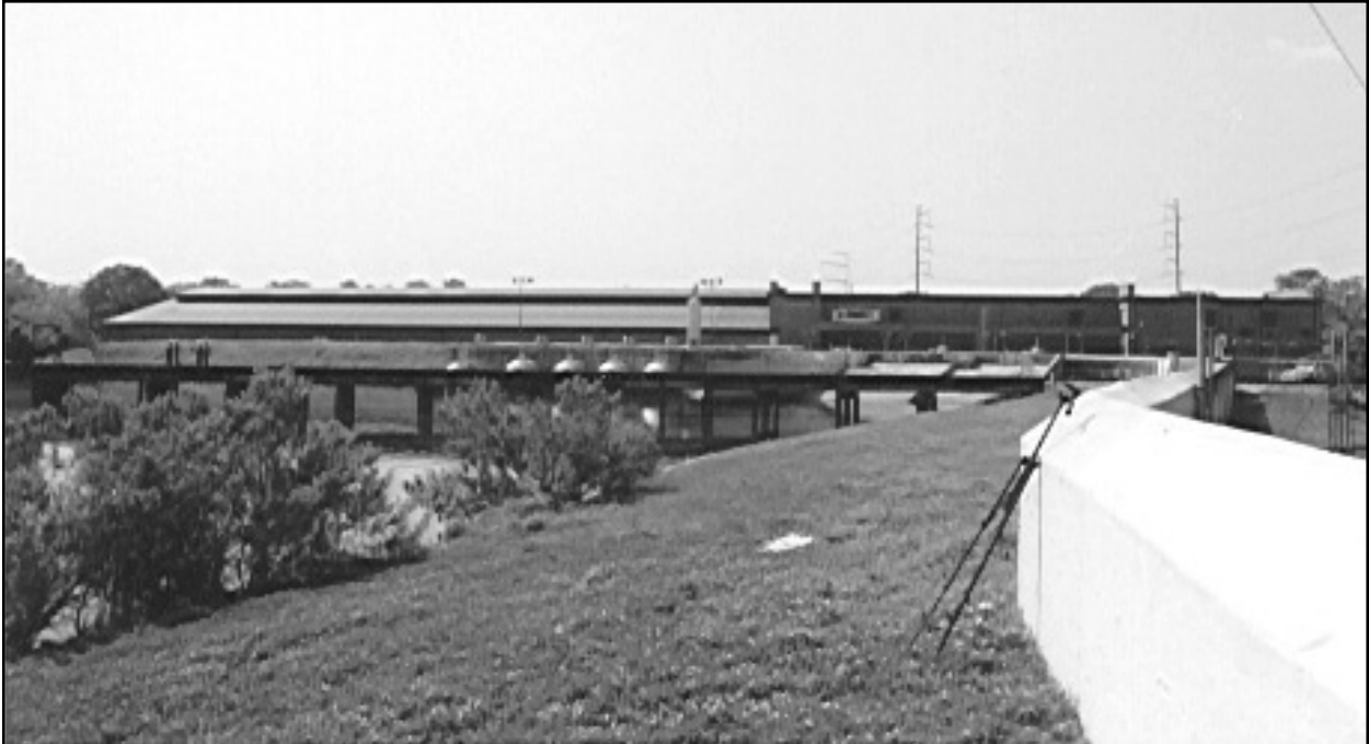
Figure 59. Drainage Pumping Station No. 6, viewed from the north.
