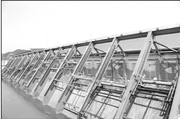
Figure 56. Drainage Pumping Station No. 6, viewed from the southwest.
