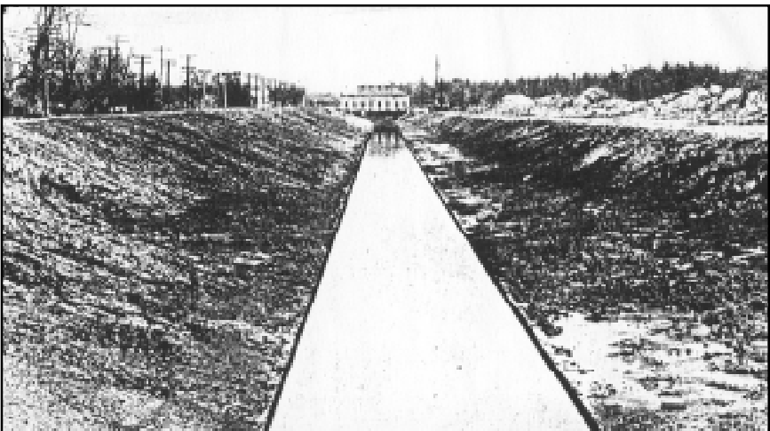
Figure 78. Lower end of the Metairie Relief Canal, approaching Pumping Station No. 6, 1914 (from Sewerage & Water Board 1914).
