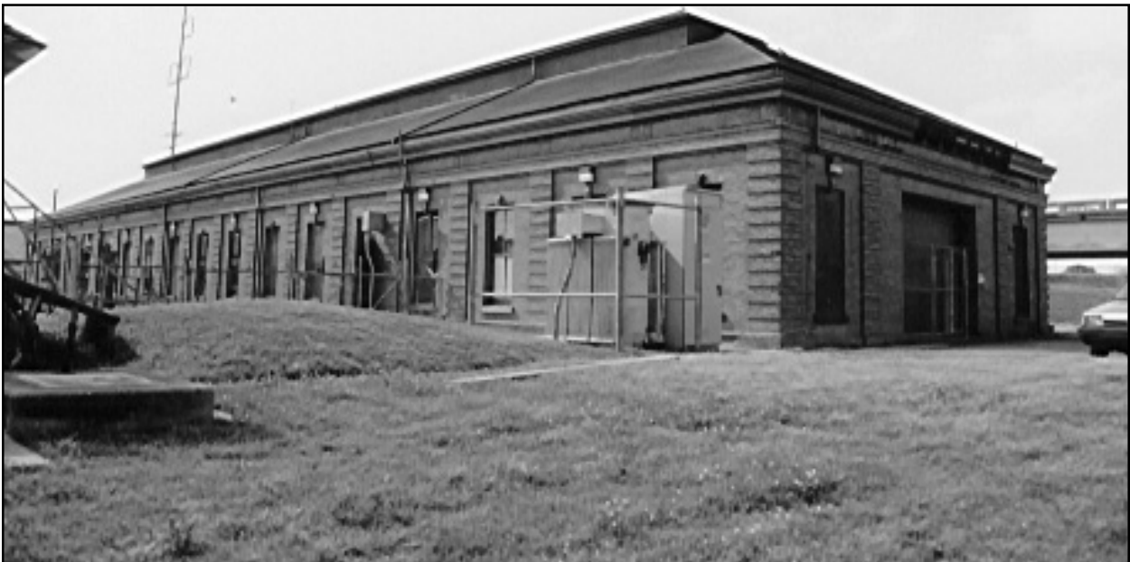
Figure 62. Drainage Pumping Station No. 7. View from the southeast.
