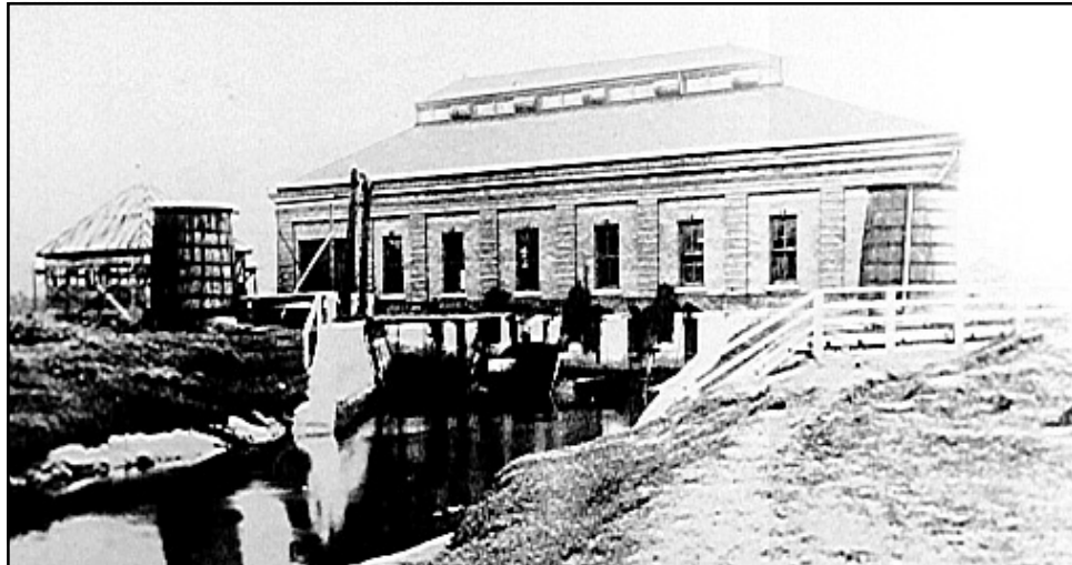
Figure 13. Drainage Pumping Station No. 1 as originally constructed, 1911 (from the Louisiana Collection, Howard-Tilton Memorial Library, Tulane University).
