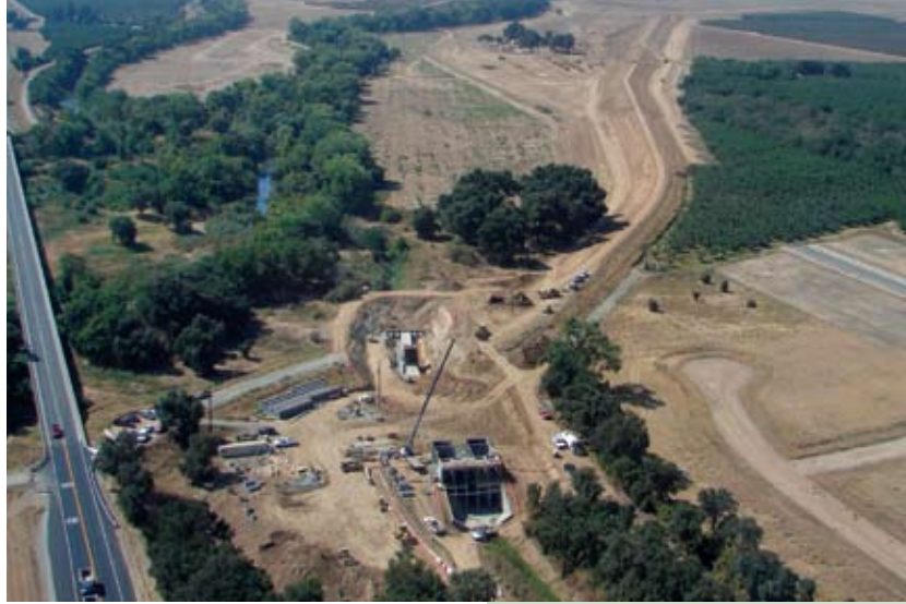
Setback levee being constructed near Bear River
