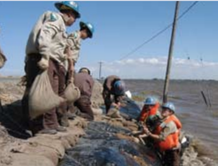
California Conservation Corps workers strengthen a levee during a high water event
