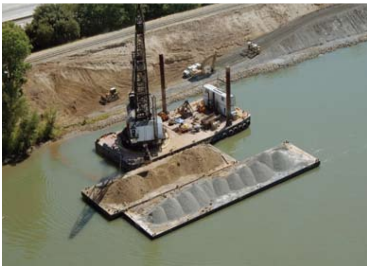
Levee repair site on Sacramento River
