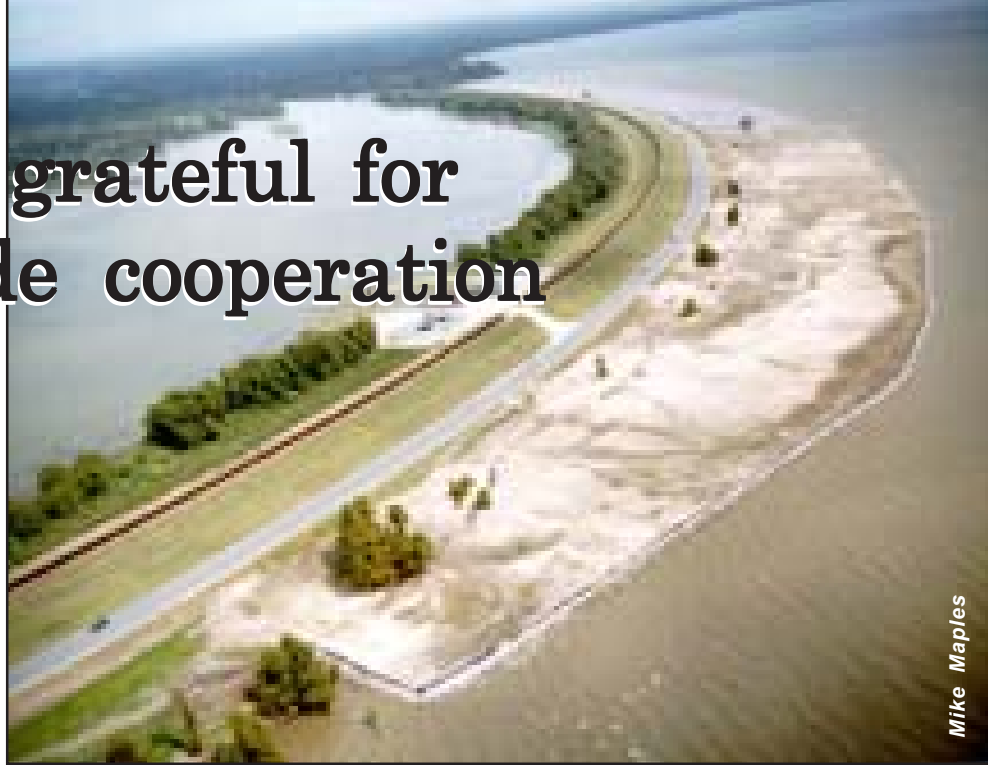
Shoreline restoration involved constructing a rock dike with dredged materials from another project in nearby Berwick Bay.
