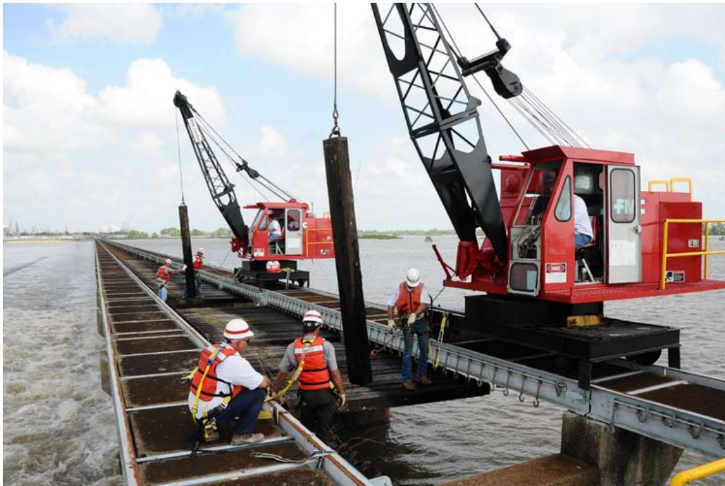
The Bonnet Carré Spillway is comprised of 350 bays, with 7,000 timber needles. A total of 160 of these bays were opened by the Corps within nine days. During the 28 days in operation, the average flow through structure was 113,000 cfs (137,000 cfs below its capacity).
