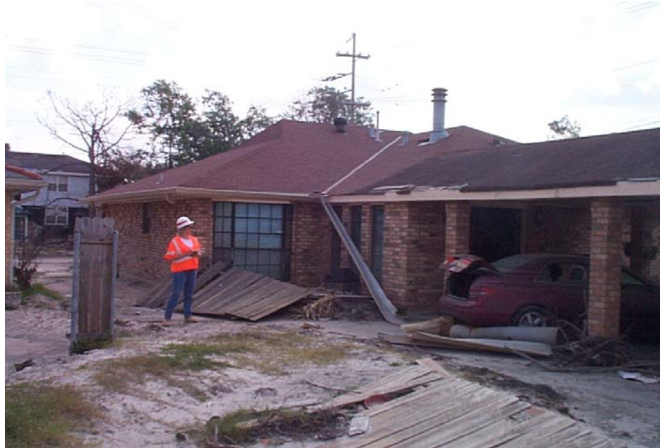
Michelle Marceaux, who is with the Corps of Engineers' Real Estate Division, measures a house on Mirabeau Ave. near the London Ave. Canal. The house was badly damaged by Hurricane Katrina. (USACE Photo)
