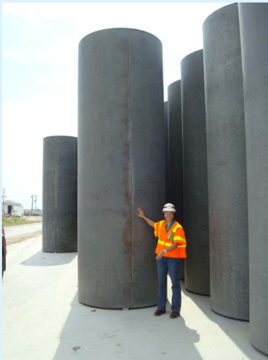
These are samples of the spun cast concrete piles that will be used in the IHNC Surge Barrier Protection project. The piles will be driven segmentally to meet the desired design depth.
