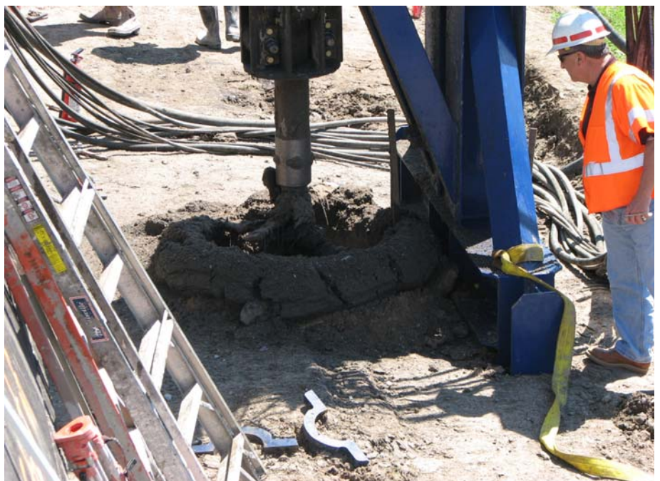
IHNC West Wall deep soil mixing to strengthen levees
