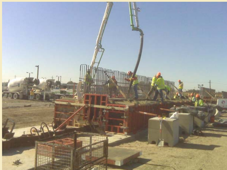
Pouring concrete for a Seabrook T-wall.
