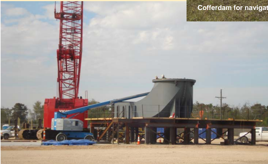
Fabrication of first pump intake
