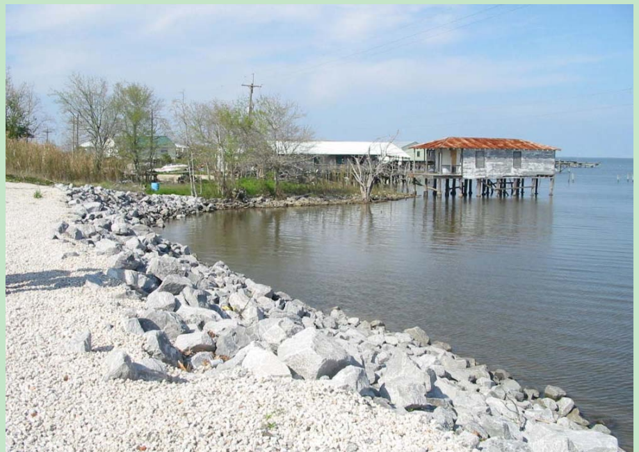
Raised houses along LA Highway 90 at Lake St. Catherine in Orleans Parish.
