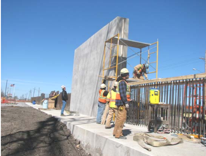
Floodwall construction on Harvey Canal
