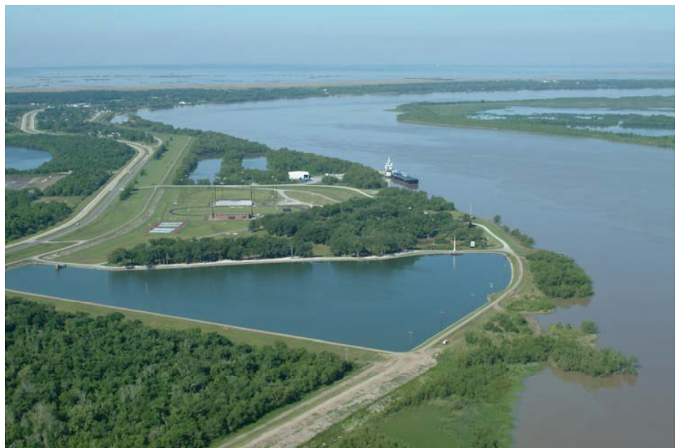
The LACPR study area includes a variety of Louisiana landscapes. Above is an aerial view of Fort Jackson on the Mississippi River in Plaquemines Parish. (USACE) Photo
