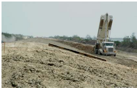
Earthen levee construction
