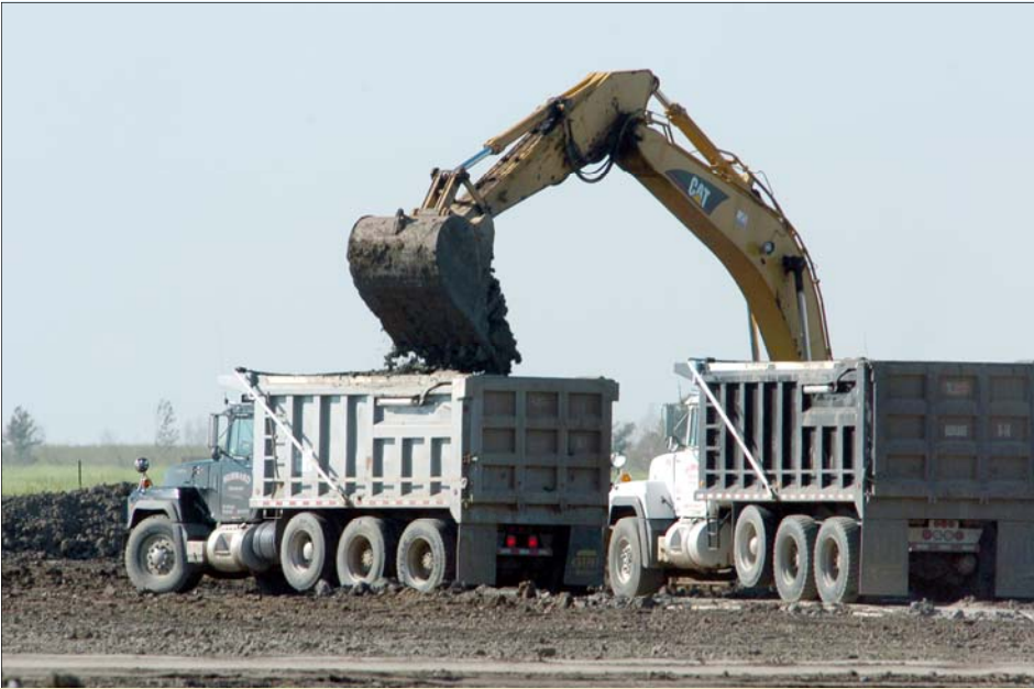
Crews excavate a large borrow pit for levee clay. (USACE Photo)
