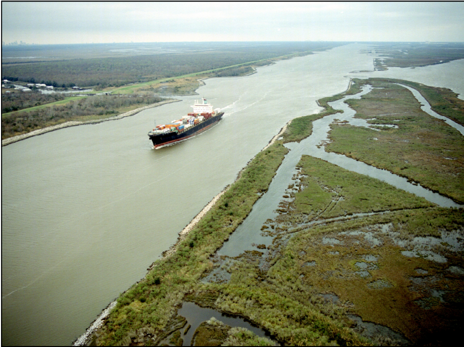
A deep draft ship navigates MRGO near mile marker 53 which is near the Bayou Dupre Control Structure. (USACE photo)
