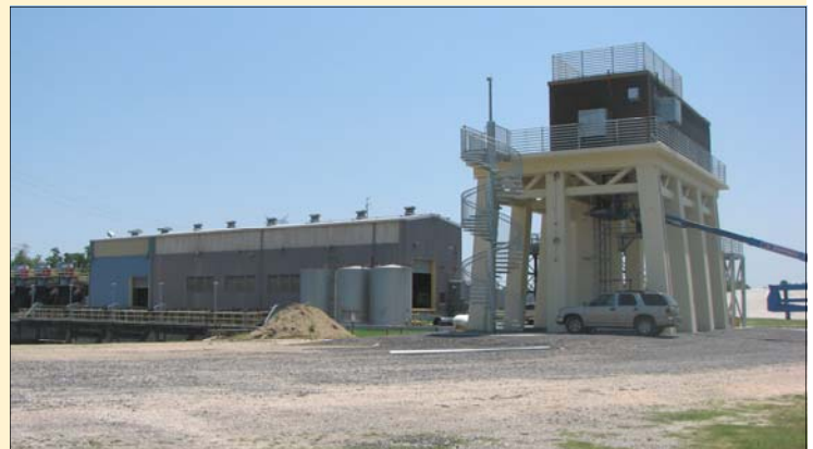
Planters Pump Station and Safe Room
