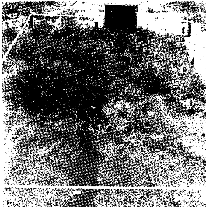
Figure 27.--Vegetation establishment; Enkamat over erodible soil; 9/29/82.
