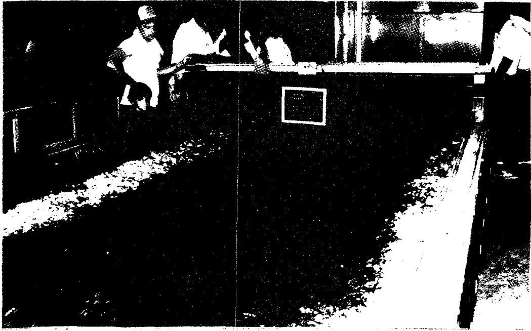
Figure 54.--Testing of loose gravel liner.
