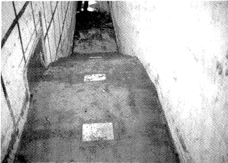
a. Looking downstream
