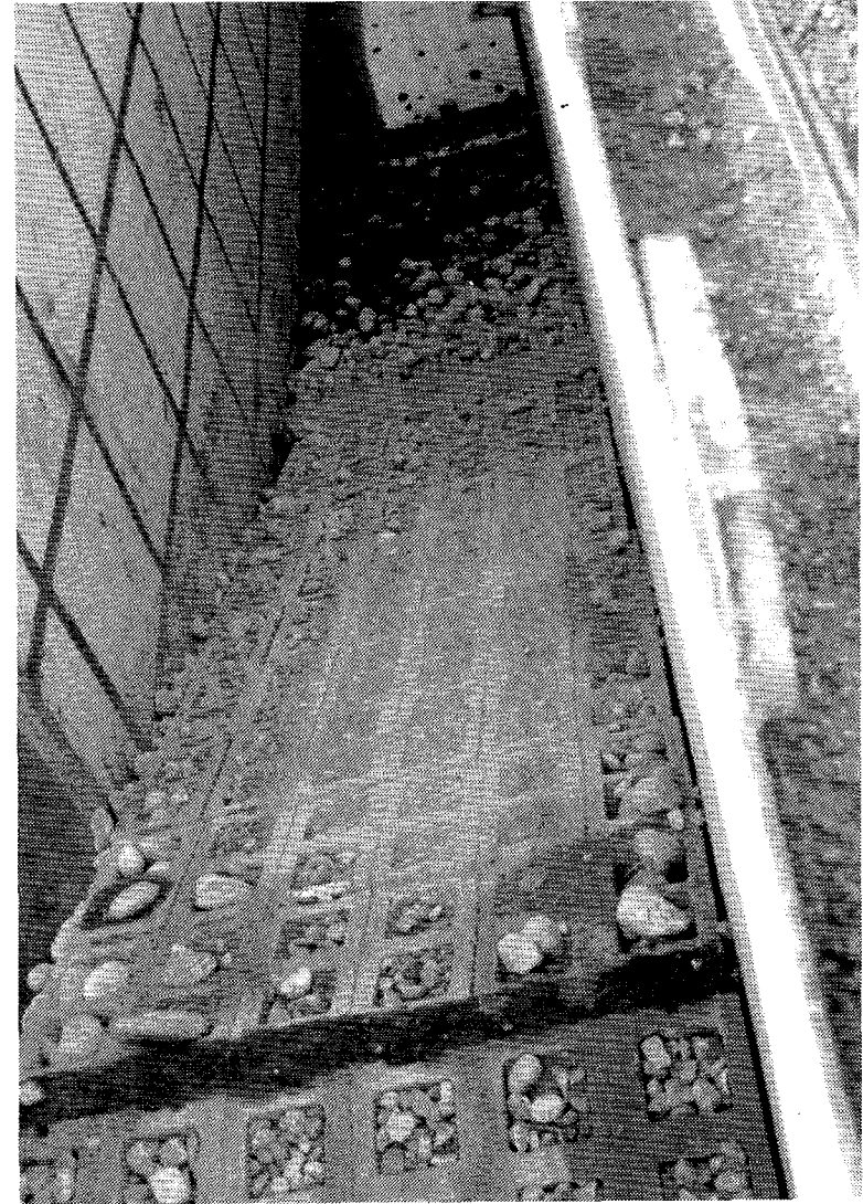
b. After placement of the gravel fill material
