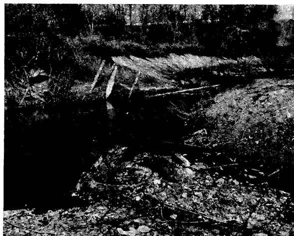
Figure 313. View in 1976 of scour hole at downstream end of concrete-lined channel
