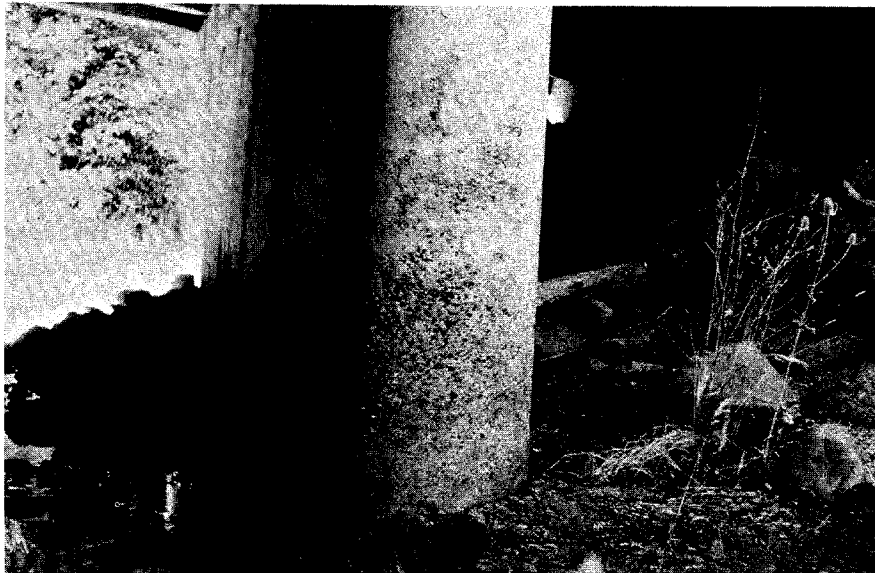
Figure 269. Abrasion damage on upstream nose of pier at right bank, Lapwai Creek, 1977.
