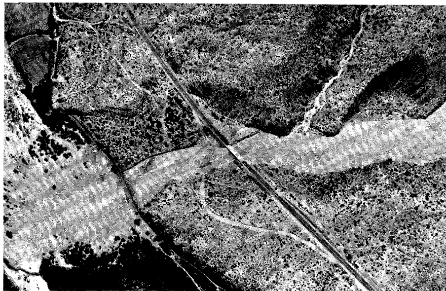
Figure 208. Aerial photograph of Bronco Creek showing channel constriction at bridge and skewness of bridge. (From Arizona Dept. of Highways.)
