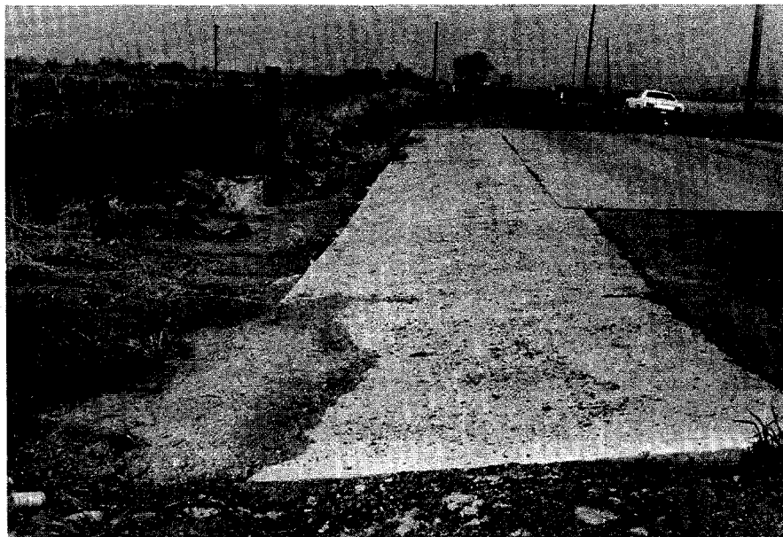
Figure 96. Concrete apron protection at downstream side of road overflow section, in 1977.
