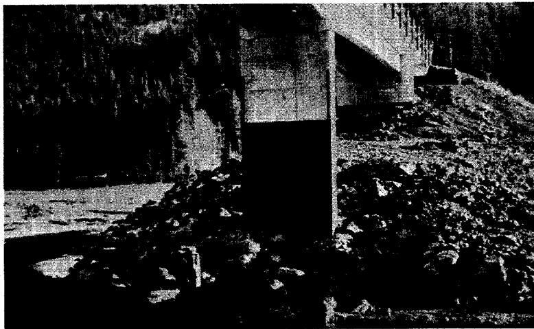
Figure 276. View of left (east) end of Lake Cushman bridge, on January 6, 1977. Footing and top seal of pier 3, center, are exposed and H-pile foundations of pier 2, background, also exposed. Note gabion wall at top of abutment fill-slope and approach alignment of stream, at left.
