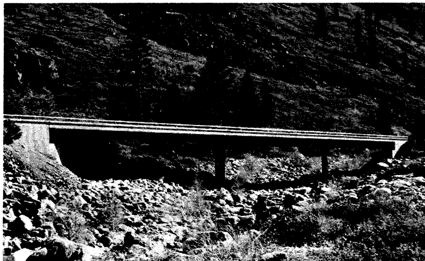
Figure 44. View downstream of Salmon Creek bridge, built in 1964.
