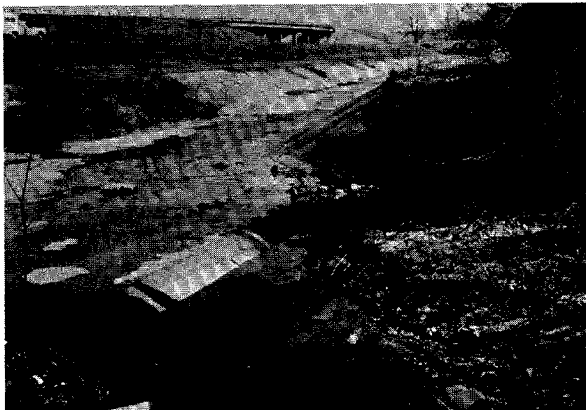
Figure 311. Upstream view of concrete-lined channel, in 1976. Concrete baffles in channel (foreground) are intended to retard flow velocity.
