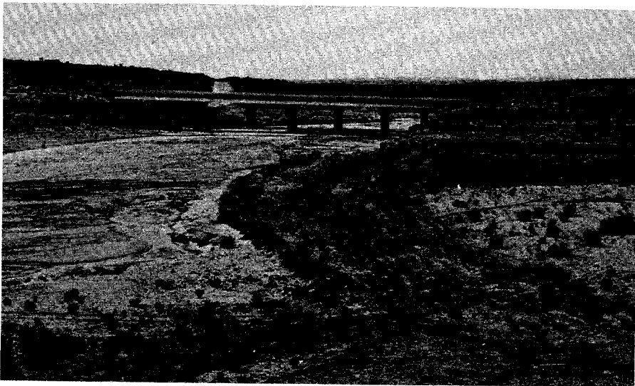
Figure 222. View of borrow pit on right-bank flood plain and damaged rock riprap protection of levee separating channel from borrow pit. (From Arizona Dept. of Highways.)
