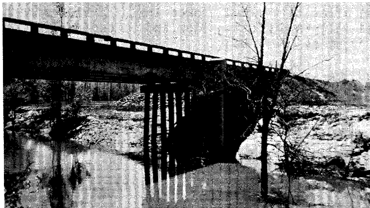
Figure 153. Upstream view of eroded left bank at bridge, on April 6, 1976, spur dike is visible beyond pile bent.
