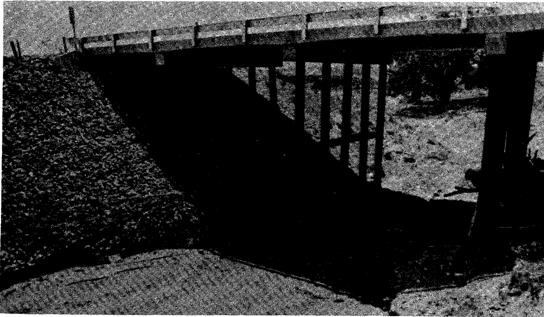
Figure 294. Upstream view of SR-192 bridge at Carpenters Draw in May, 1977, showing rock-and-wire mattress on abutment fill-slope, left, which extends to center of channel. Mattress on opposite slope also extends to center of channel. At lower left, wire is failing to hold riprap.
