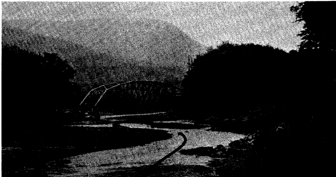
Figure 238. Upstream view of bridge and spurs, US-15 near Covington, PA.
