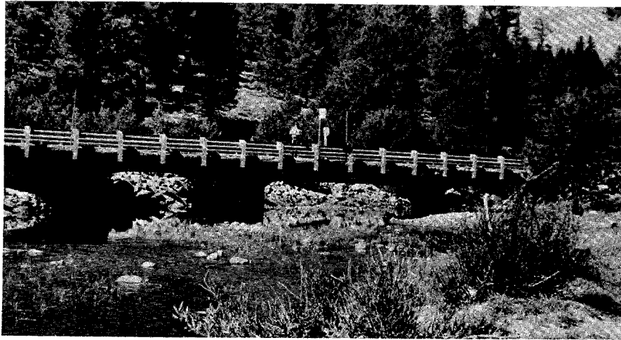
Figure 74. View upstream, in 1976, showing clearance of bridge at time of low flow.
