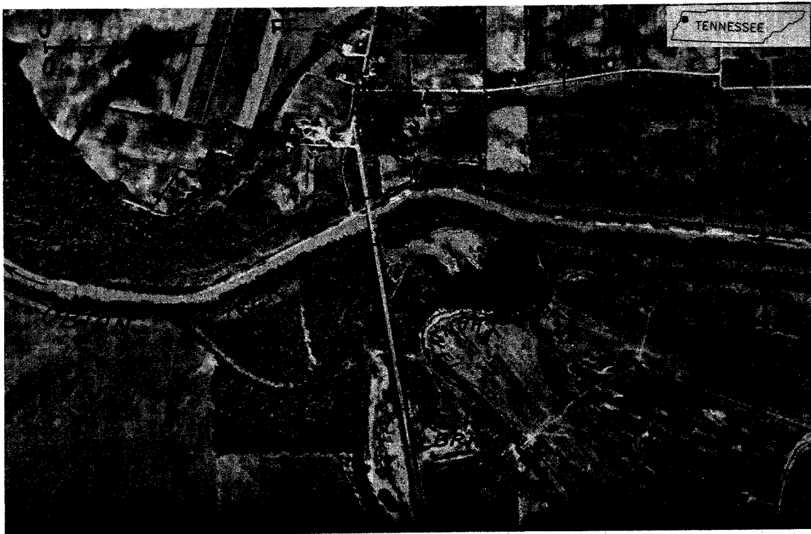
Figure 258. Vertical aerial photograph of Obion River at S-8005 bridge, on November 3, 1971, just prior to bridge failure. (From U.S. Dept. of Agriculture.)
