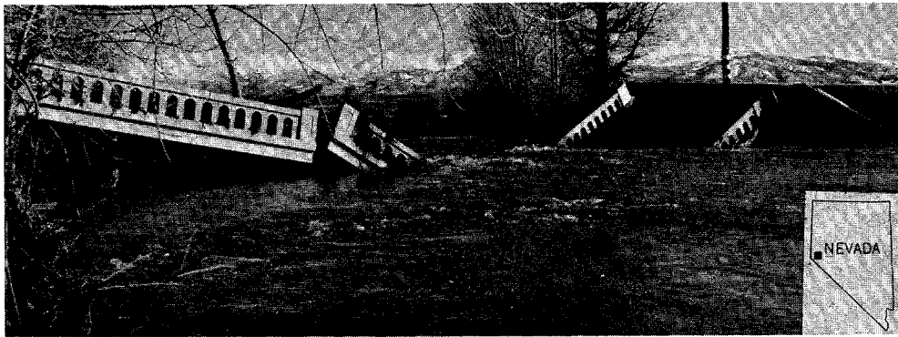
Figure 128. Failure of piers founded on spread footings, during Dec. 1955 flood. (From Nevada Dept. of Highways.)
