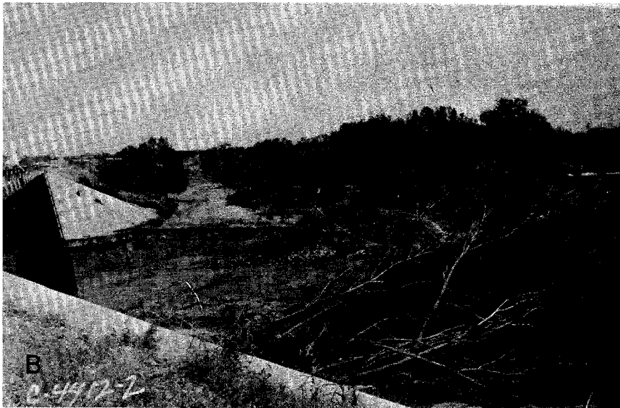
Figure 319. Undermining of concrete slope pavement during flood from Hurricane Beulah, 1967. A, upstream side of bridge; B, downstream side of bridge. (From Texas Dept. of Highways).
