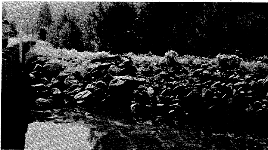
Figure 76. Heavy rock riprap on upstream right-bank dike, in 1976.
