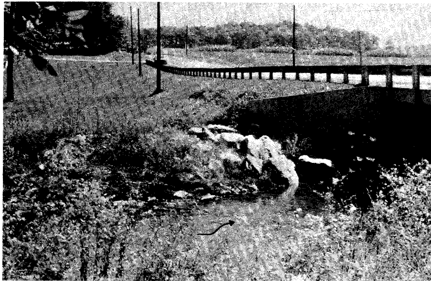
Figure 273. View of rock riprap placed on bank upstream from box culvert entrance to prevent lateral erosion when flows on the left-bank flood plain enter the main channel.
