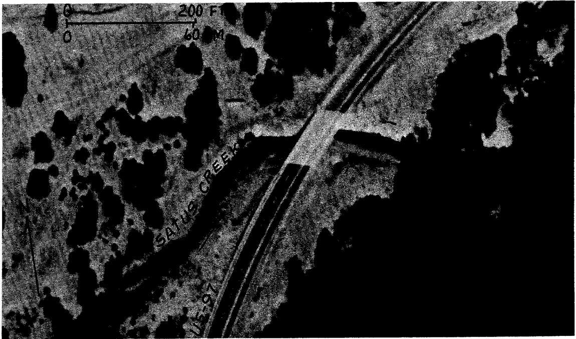
Figure 286. Aerial photograph of fifth crossing of Satus Creek, prior to flood damage. (From Washington Dept. of Highways, 1966.)
