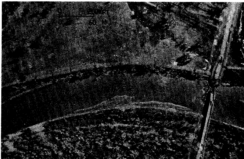
Figure 208. Aerial photograph, taken March 29, 1971, showing failure of bridge and location of spurs on left bank upstream from bridge. (Nebraska Dept. of Roads photograph.)
