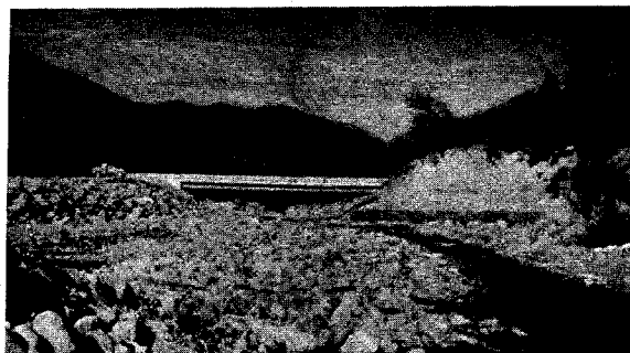
Figure 245. View downstream towards bridge showing completed countermeasures, 1977.
