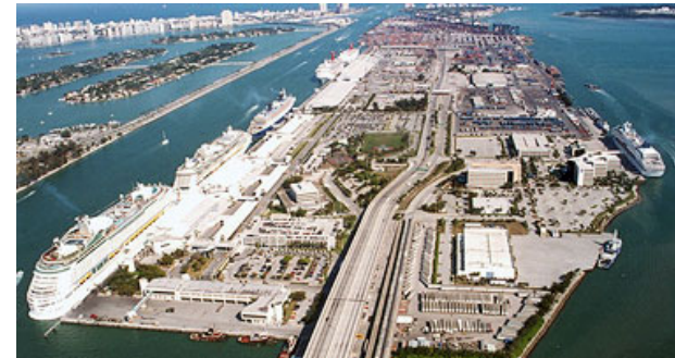
Port of Miami Tunnel, FL
