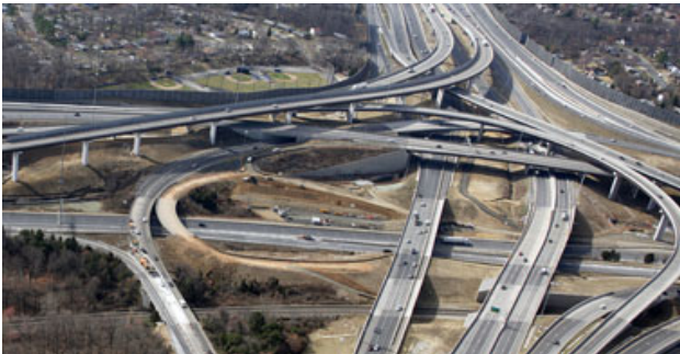
Capital Beltway, HOT Lanes, VA
