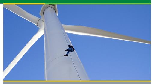
Modern, three-blade wind turbines are 50 to 90 meters in diameter and are mounted atop towers that stand 60 to 100 meters high. Typically, towers are installed in arrays of 30 to 150 machines.
