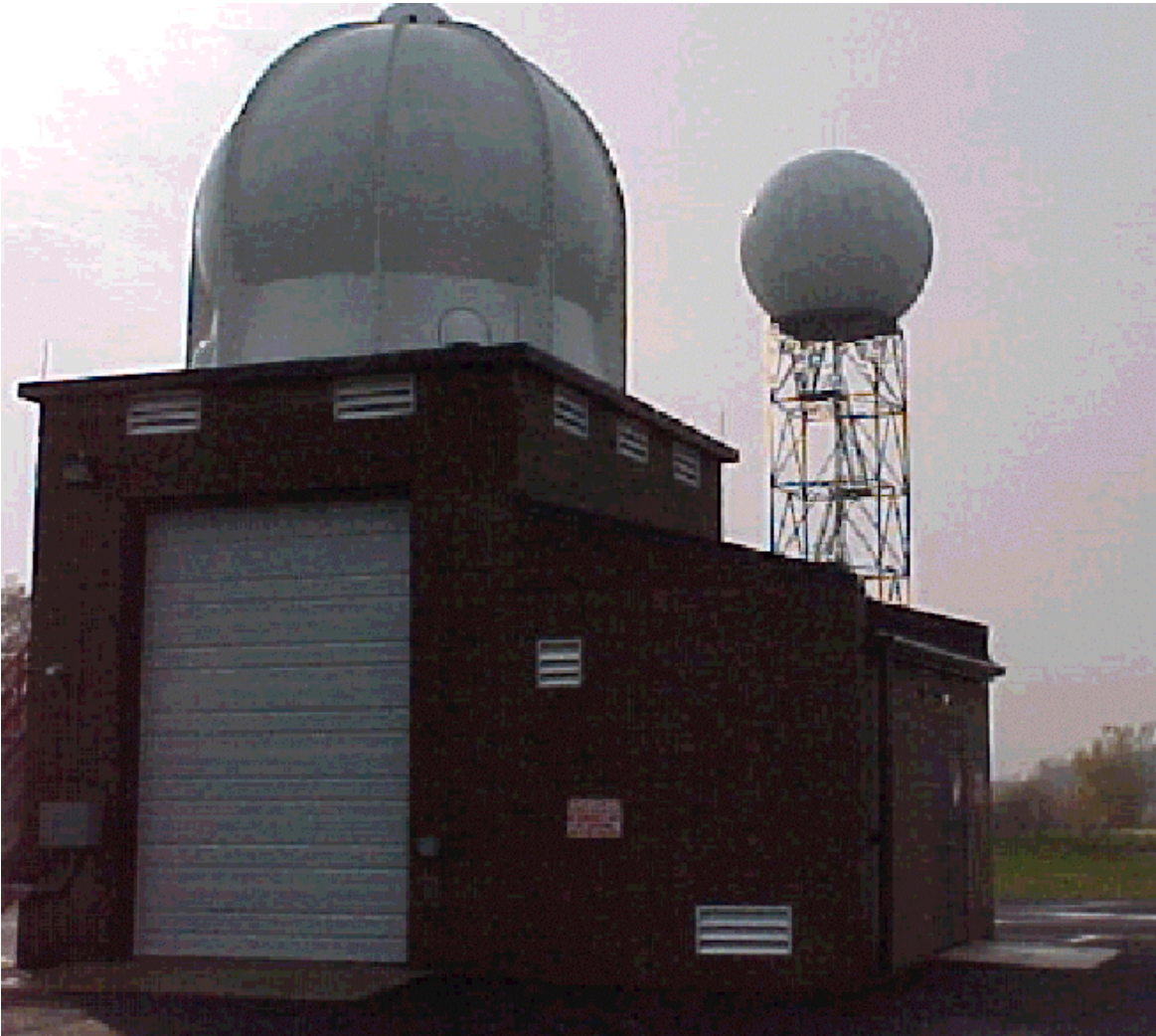
Figure B-2 - NWS Low-Bay Upper Air Shelter
