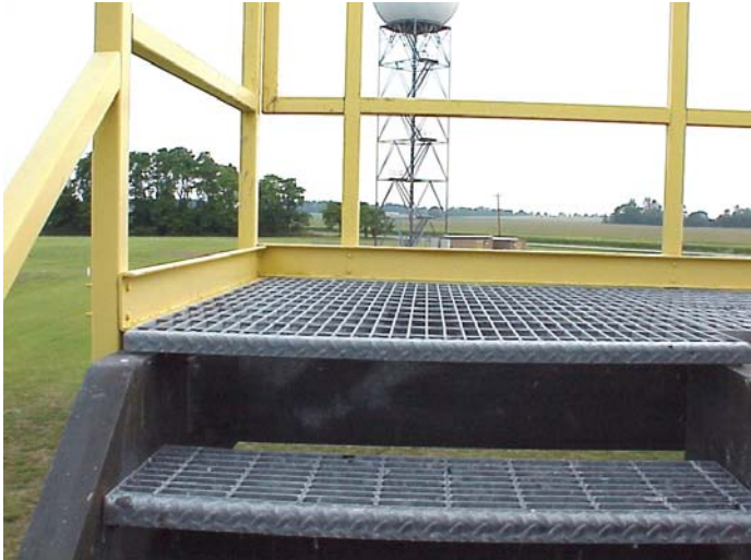
Figure K-9 - Foot Plate at Top of Stairs
