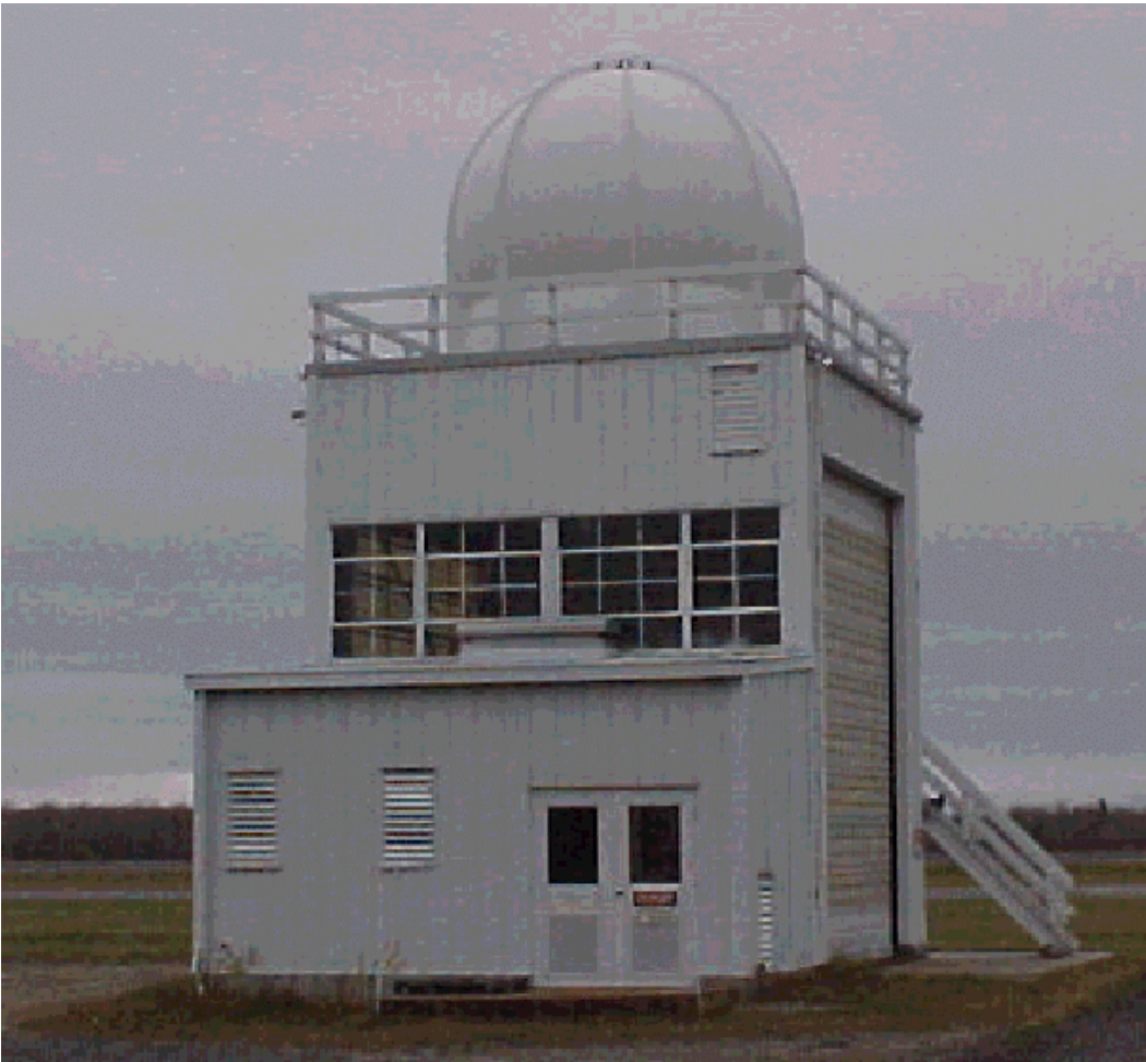
Figure B-1 - NWS High-Bay Upper Air Shelter
