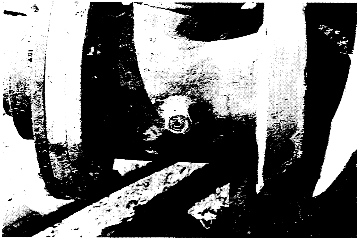
Figure 21: Close-up views of the end of the shaft shown in Figure 20.
