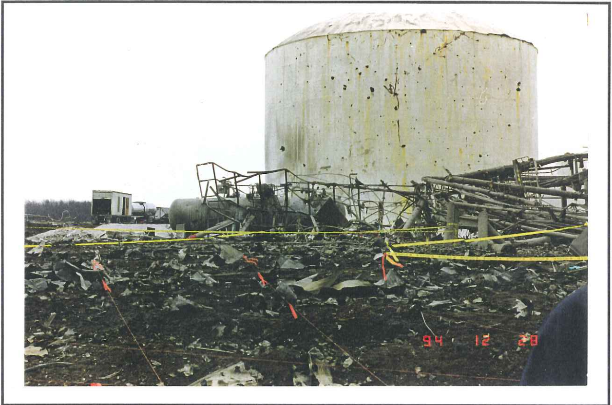
Photo 8 - 12 Water Tank Damage (Ammonia Tank Background)
