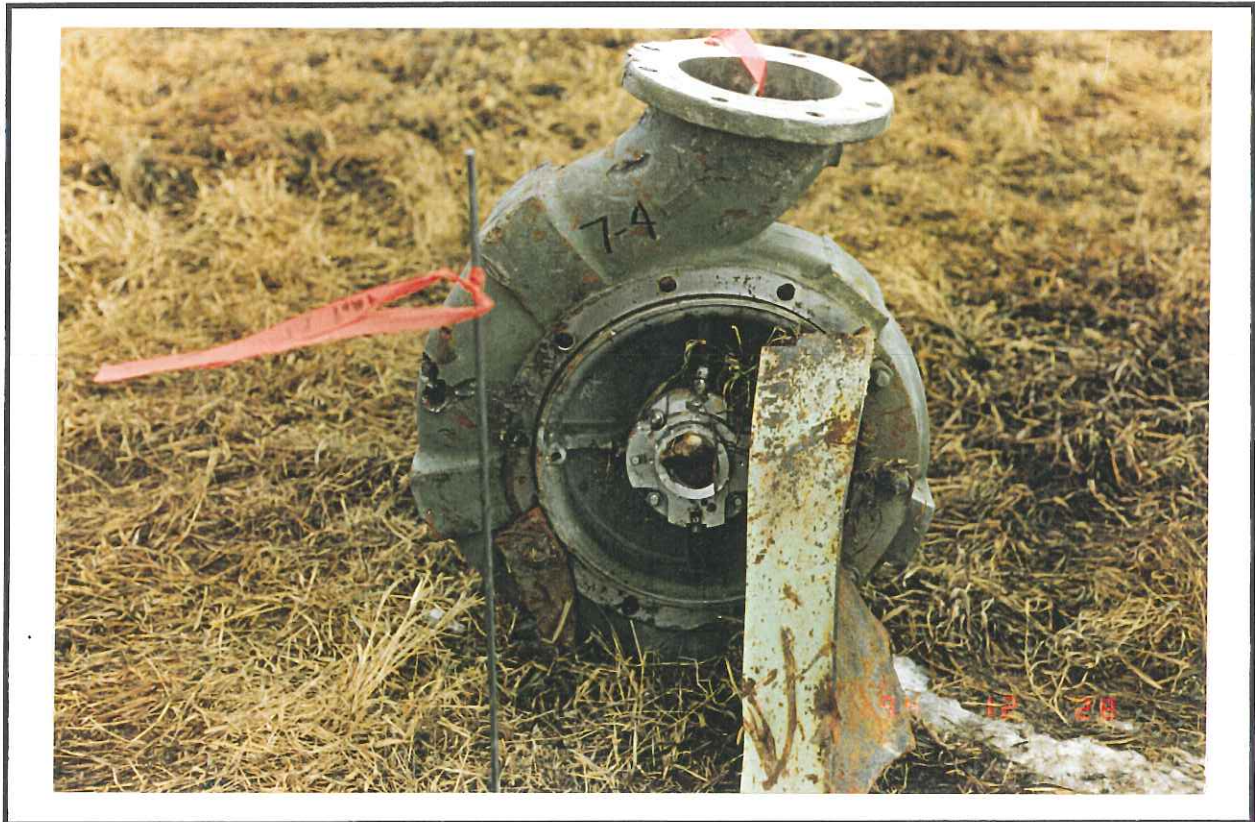
Photo 8 - 4A 416J Shaft View
