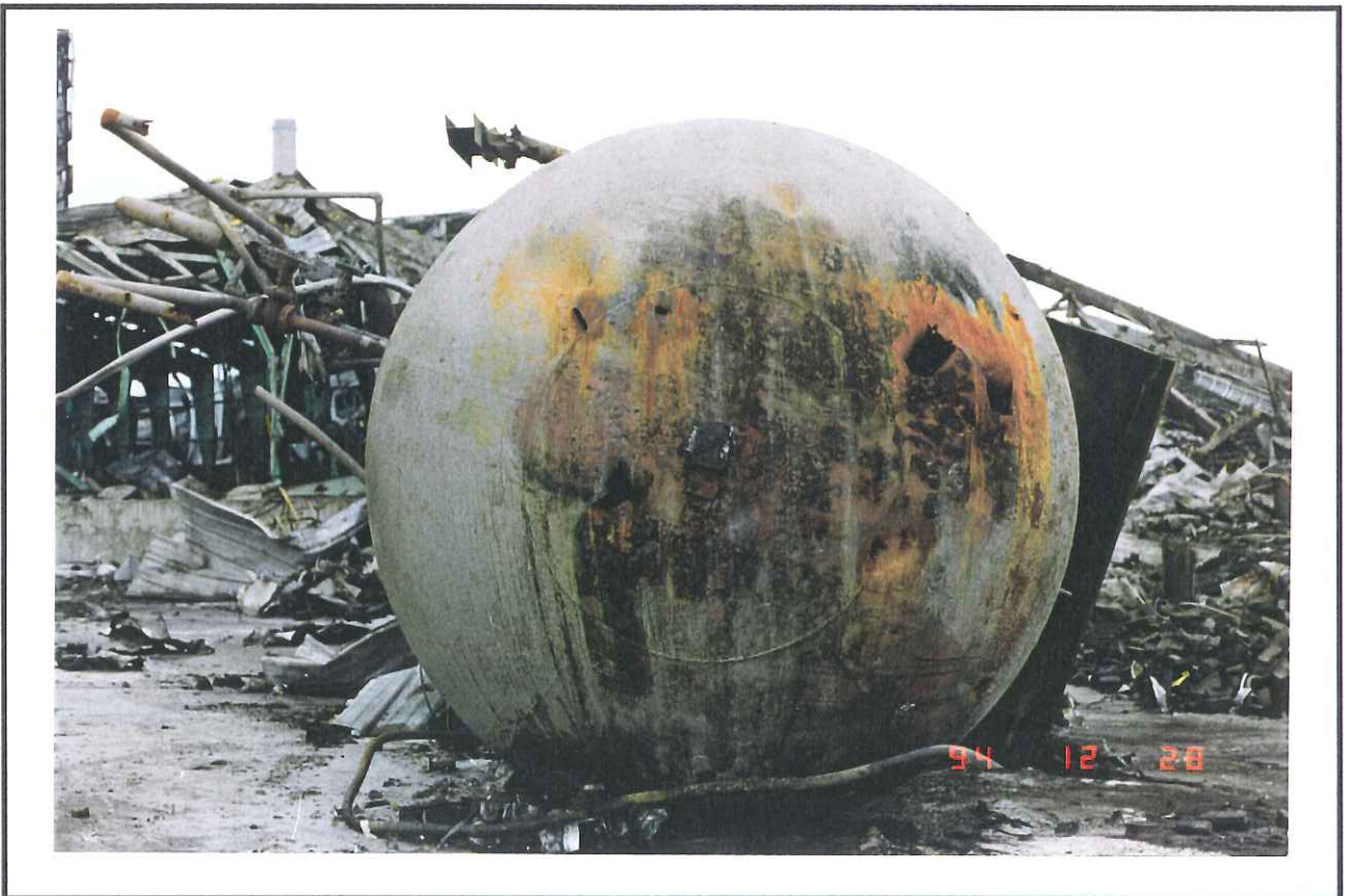
Photo 8 - 13 Ammonia Bullet Tank Damage
