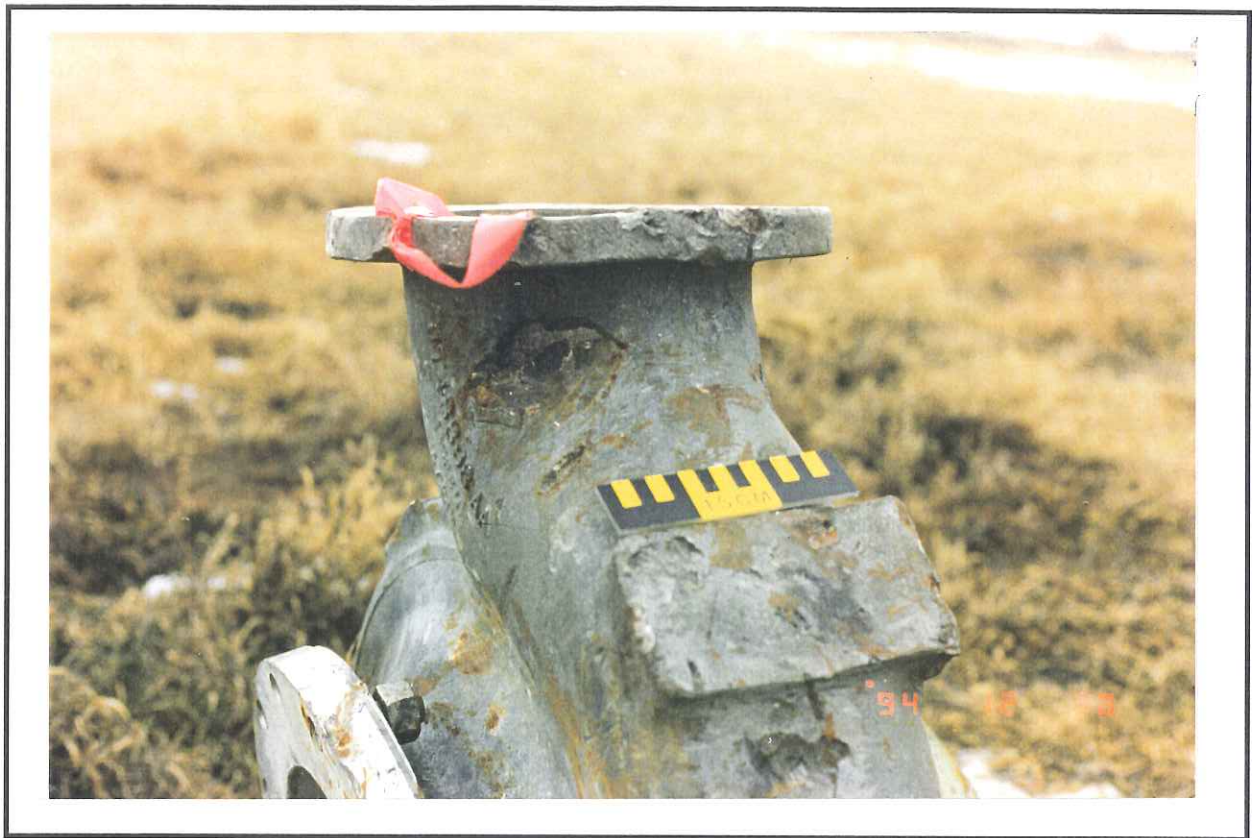
Photo 8 - 5 416J External Damage
