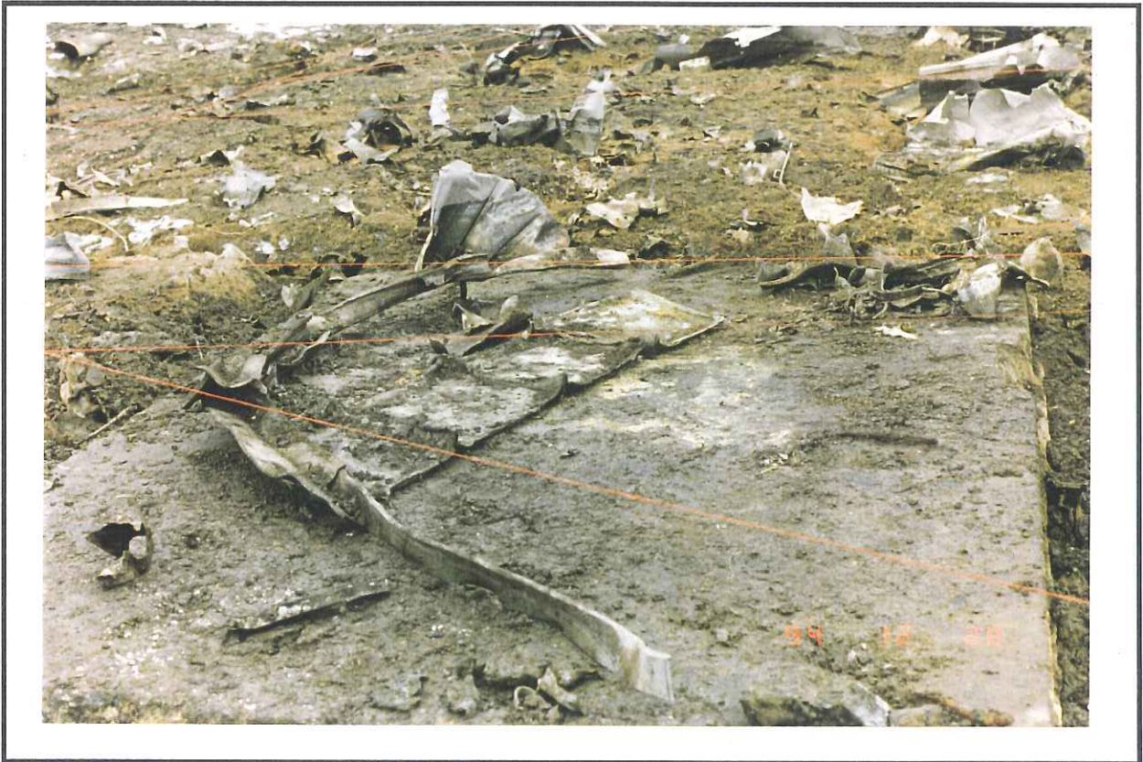
Photo 8 - 3 AN Scrubber Pad and Vessel Floor
