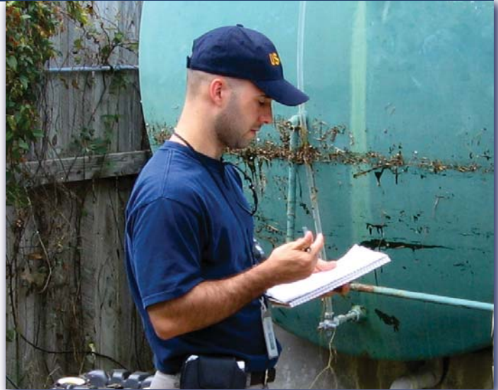
Field Inspection of an Above Ground Storage Tank
