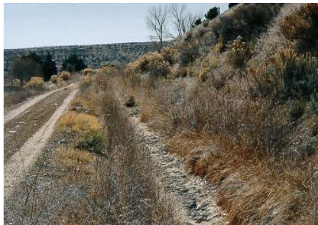
Figure 20 - Unimproved Canal at Hammond Project.
