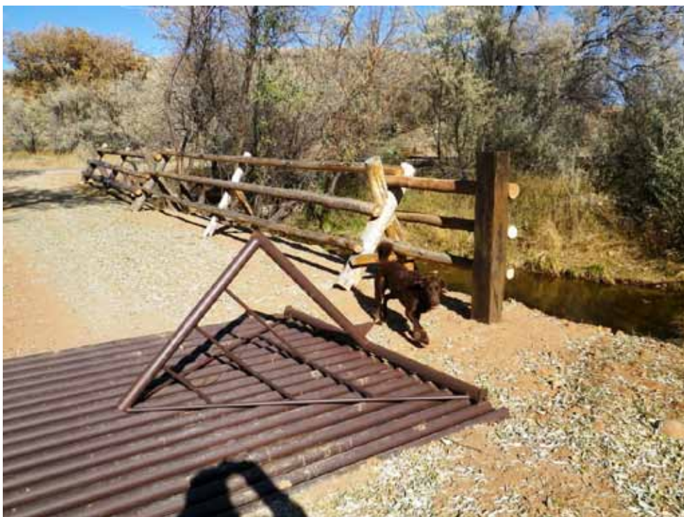
Figure 48. November 15 2011, cattleguard installed with ingenious horse gate
