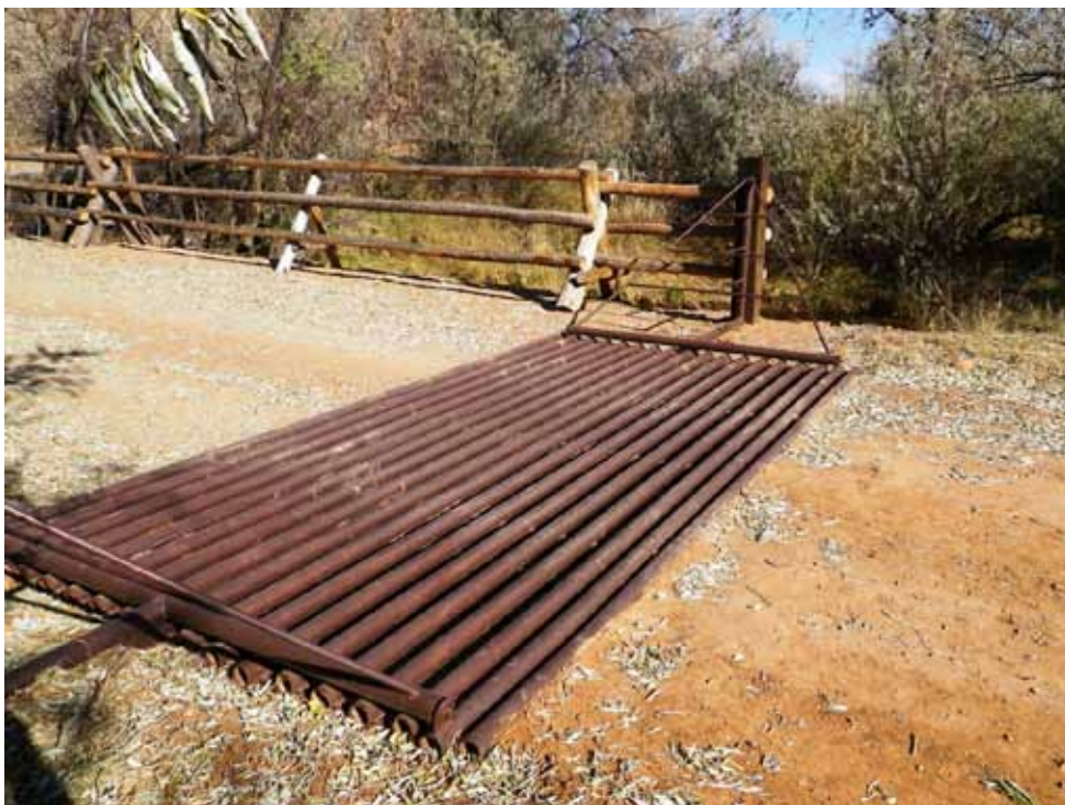
Figure 47. November 15 2011, cattleguard installed with ingenious horse gate
