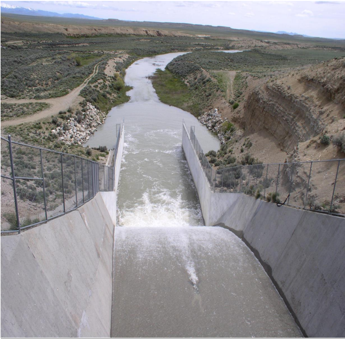
Spillway of the Big Sandy Reservoir
