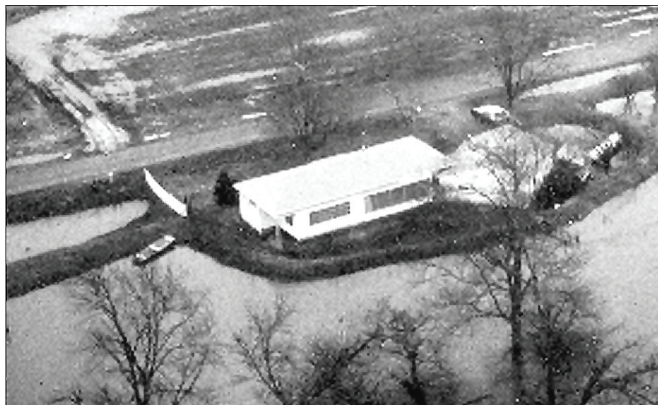
Figure 3-11. A home protected by a levee, which holds back the floodwaters shown in the lower half of the photograph. Note that the levee ties in to high ground created by the road embankment.
