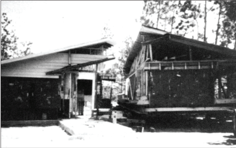
Figure 7-1. When a home is too large to be moved in one piece, it may have to be cut into sections that can be moved separately and then reassembled at the new site.
