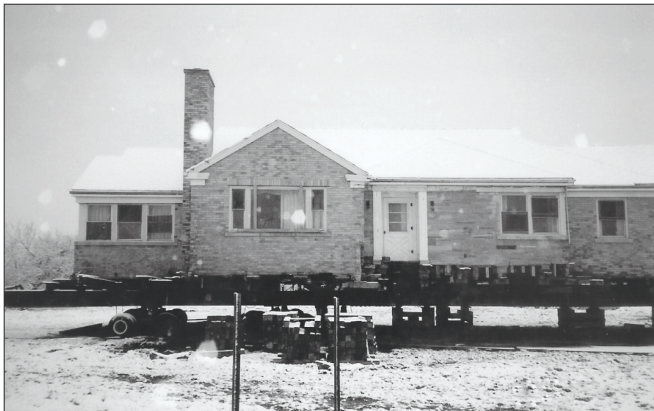
Figure 7-3. The move to the new site begins.
