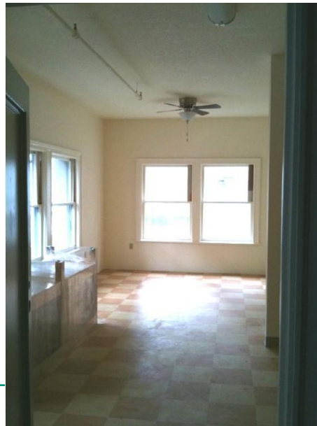
Interior of Martha Washington unit, nearing the completion of renovation. When completed, modern appliances will be energy efficient, giving way to LEED certification
