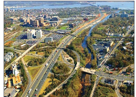
Capital Beltway high-occupancy toll lanes was the first project to utilize PABs.
