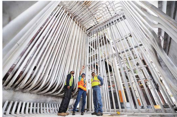
Inspecting a heater constructed under the Heating Systems Modernization project at Sandia National Laboratories.
