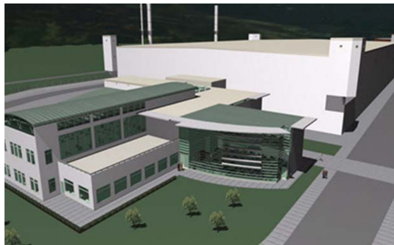
The proposed Uranium Processing Facility will ensure NNSA's long-term capability to safely and securely manage existing highly enriched uranium inventories to meet mission requirements.
