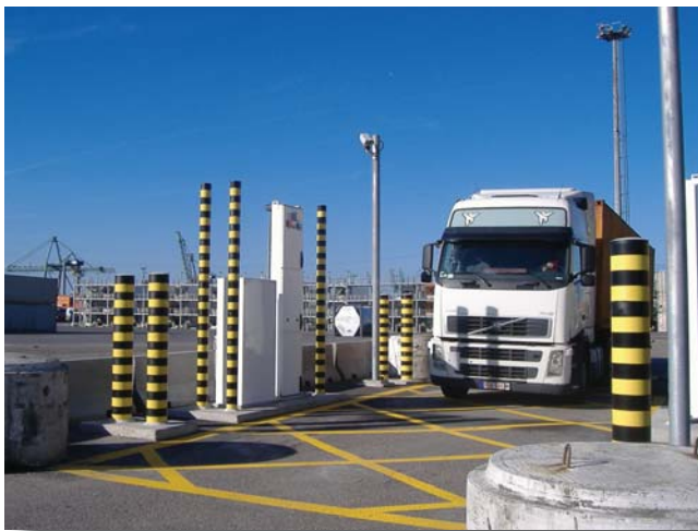
NNSA’s Megaports Initiative portal monitors at Antwerp in Belgium detect illicit trafficking of nuclear and radiological material.
