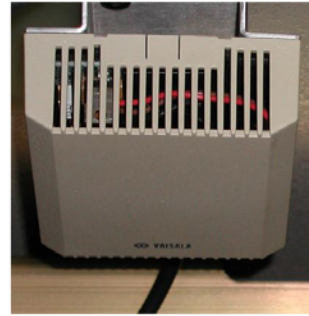
Figure 19. Humidity sensor.
