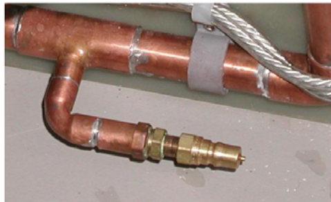
Figure 7. Quadrant water drain port
