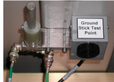
Figure 25. Typical test point located at top-center in each quadrant.
