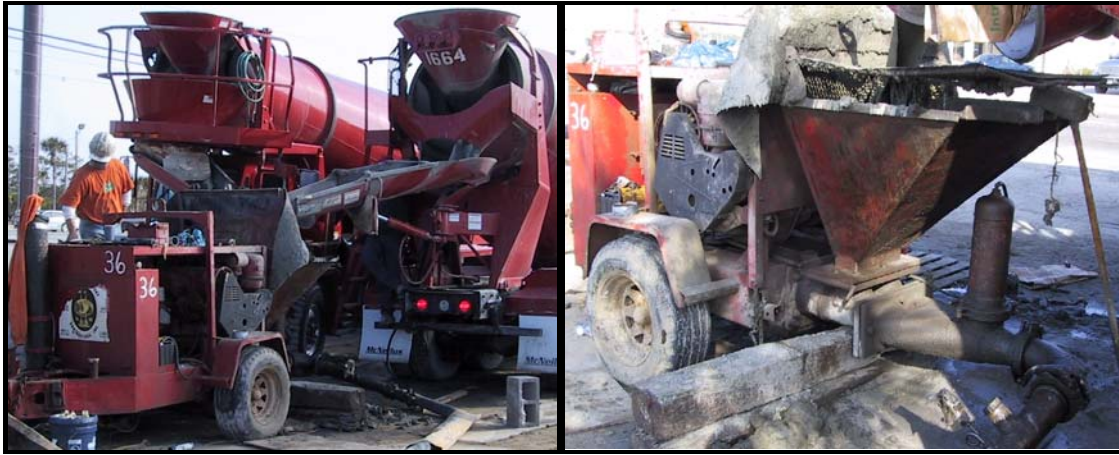
(a) Trucks Discharging into Pump
