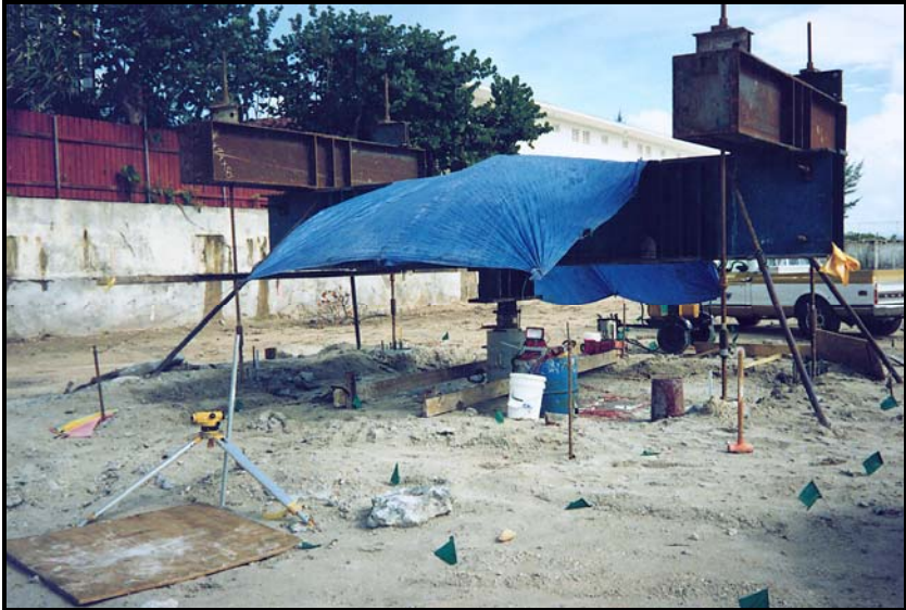
Figure 7.15: Static Load Test Setup on CFA Piles
