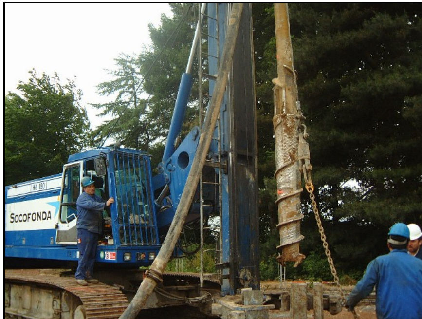
Figure 4.12: Omega Screw Pile
