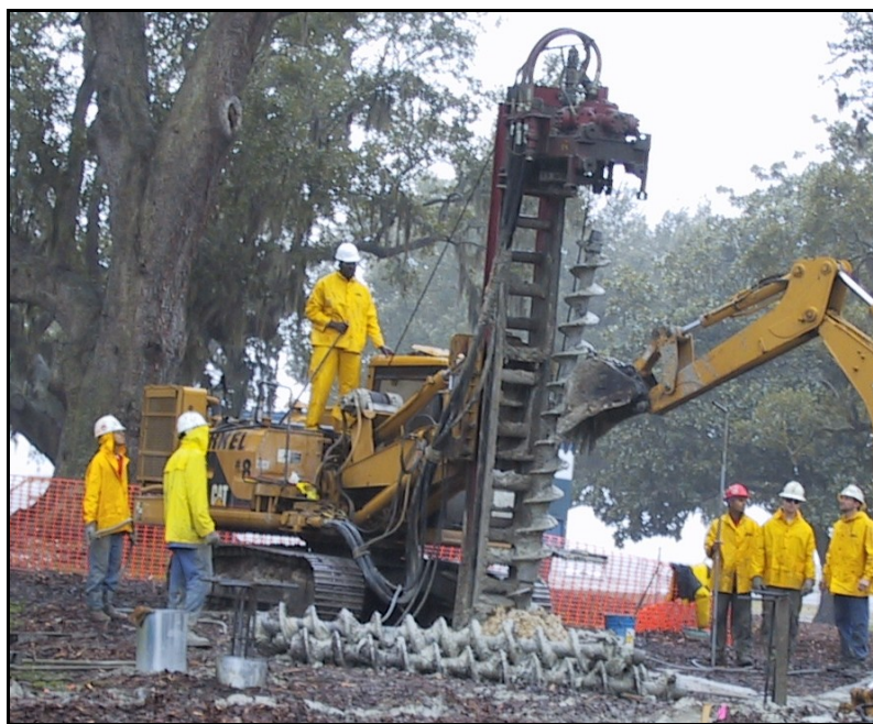
Figure 4.4: Low Headroom Rig with Segmental Augers
