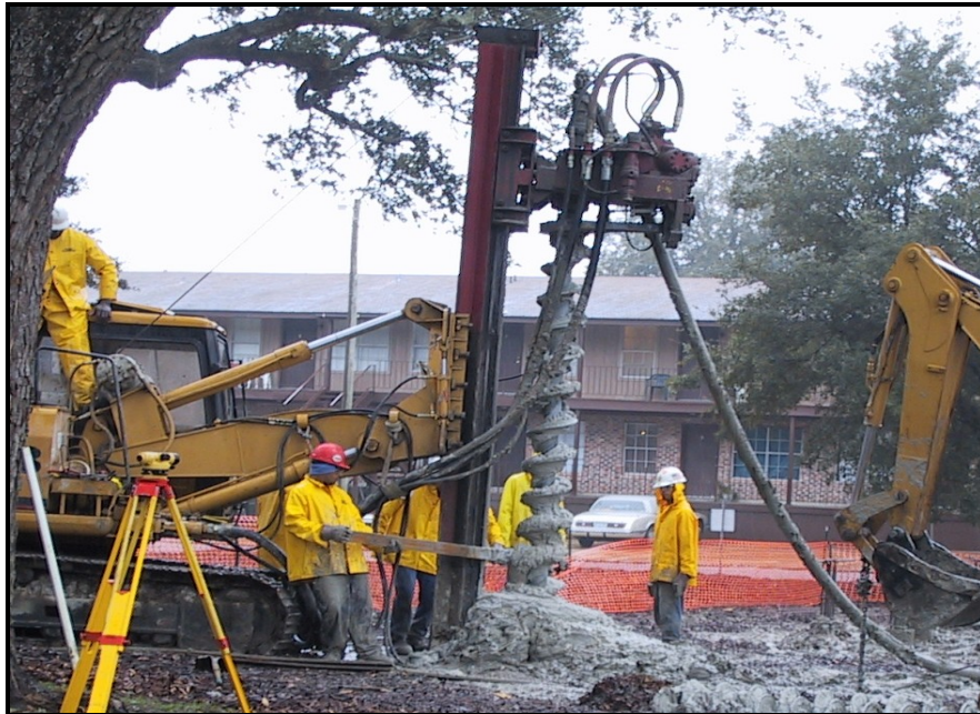
Figure 3.4: Low Headroom CFA Pile Application
