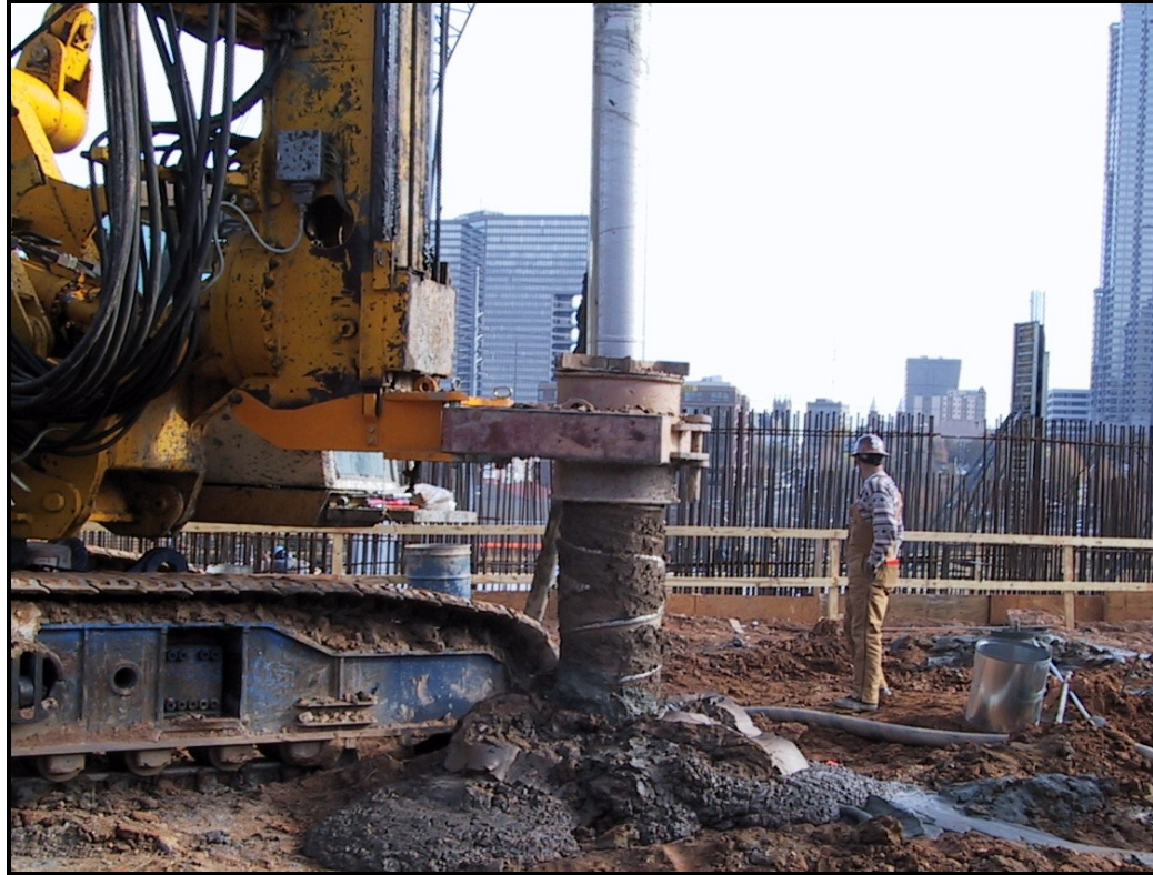
Figure 3.8: Drilled Displacement Piles Limit Spoil Removal
