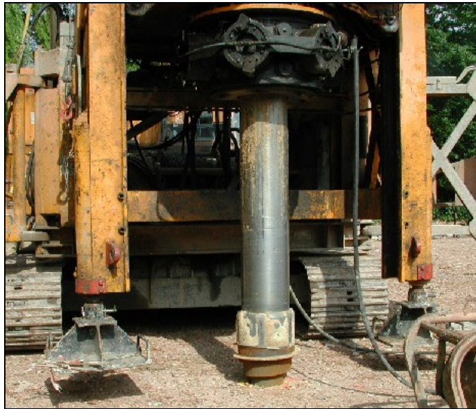
Figure 4.13: Fundex Screw Pile
