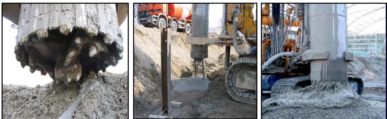
(a) Cutting Head (b) Concrete Placement (c) Cuttings Discharge
