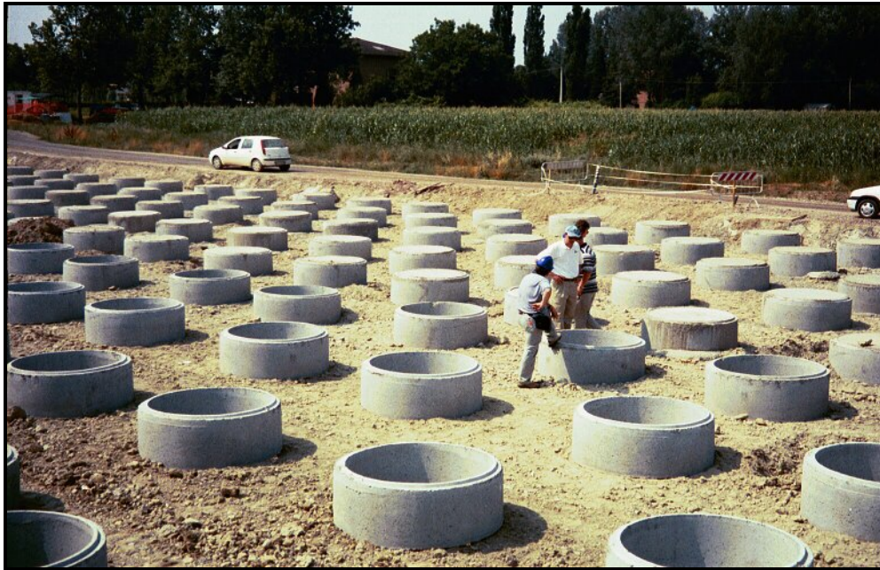
Figure 3.7: Pilecaps on CFA Piles for a Pile-Supported Embankment
