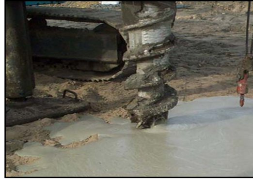
Figure 2.9: Grout at Surface after Auger Withdrawal
