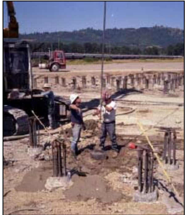
Figure 2.11: Placement of a Single Full-Length Bar
