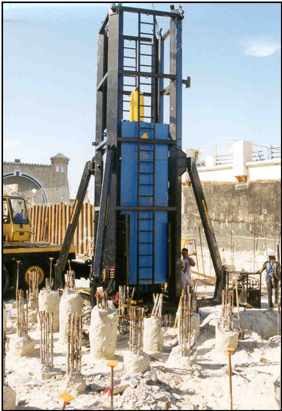
Figure 7.16: Proof Testing of Production Piles with Statnamic (RLT) Device
