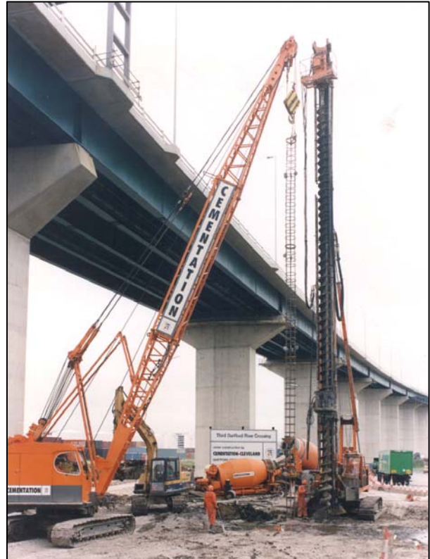
Figure 3.3: CFA Piles at Bridge Interchange
