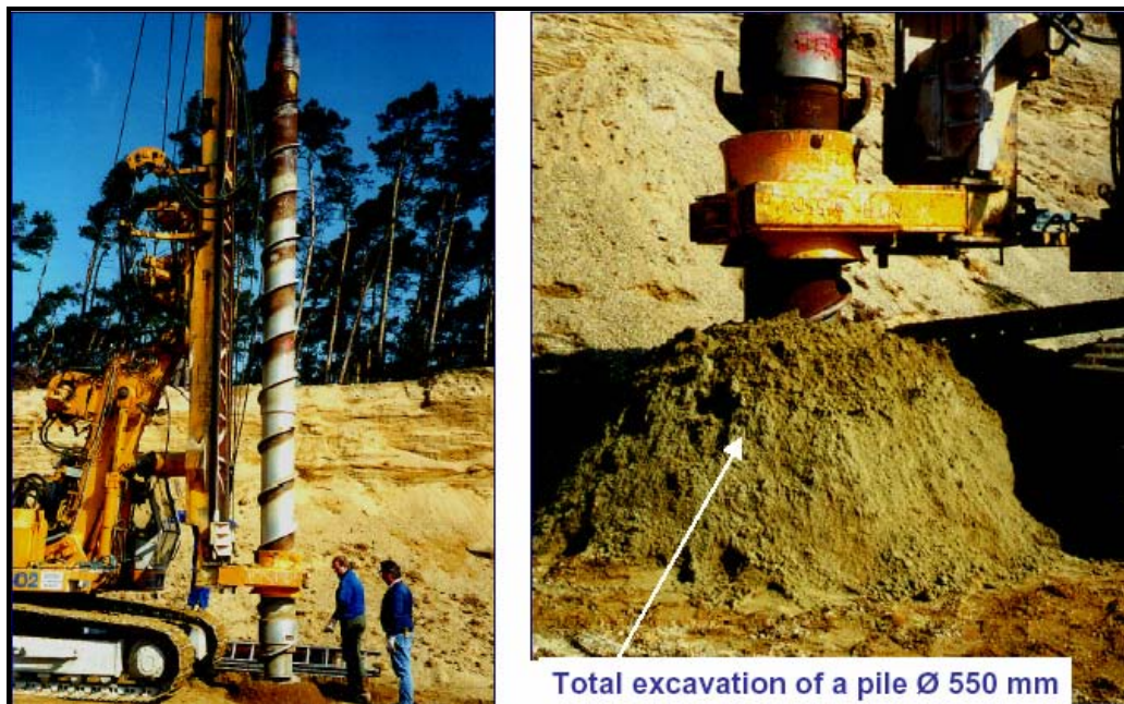
(b) Partial Displacement Auger
