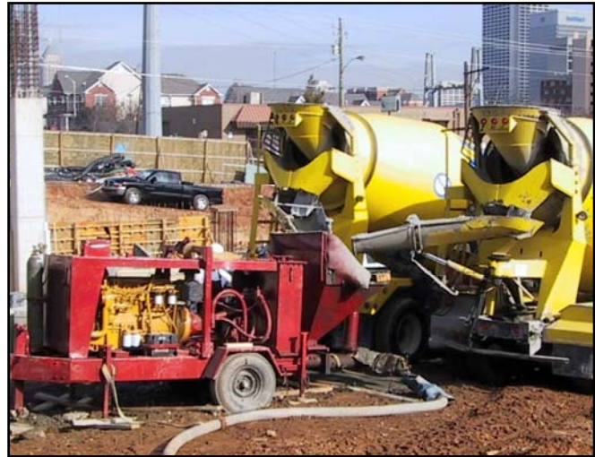
Figure 2.8: Grout Delivered to Pump
