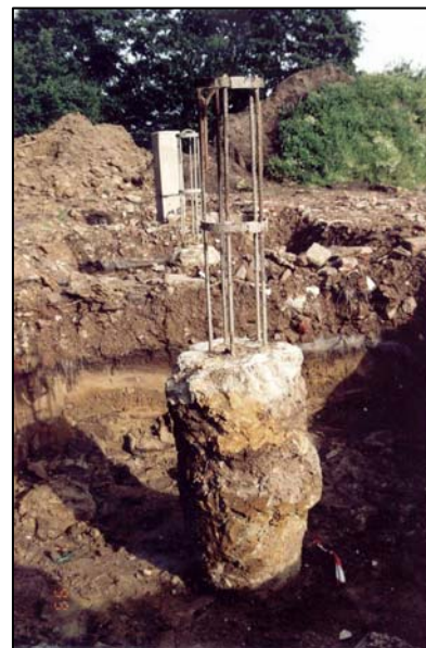
Figure 4.13: Fundex Screw Pile
