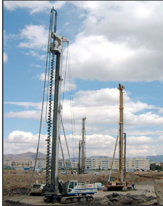
Figure 4.6: Soilmec Hydraulic CFA Rig with Kelly-Bar Extension
