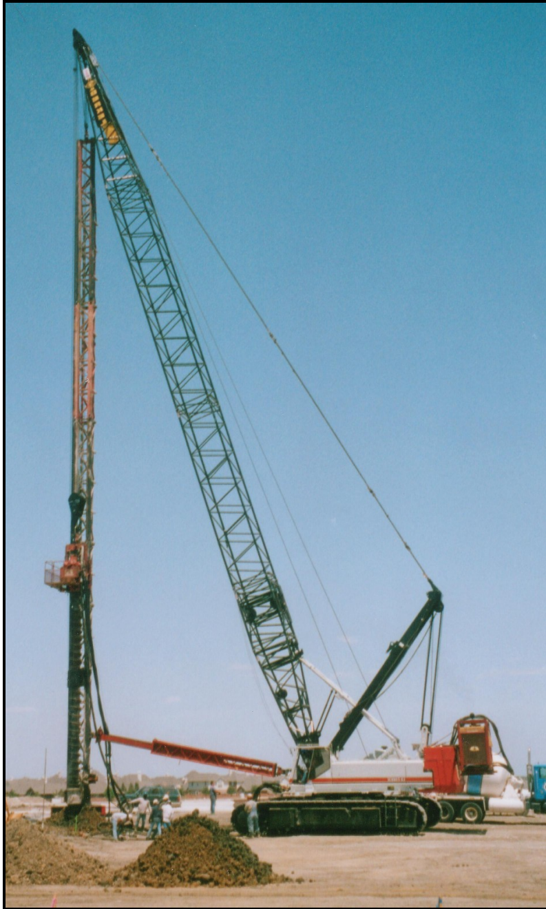
Figure 4.2: Photo of Crane-Attached CFA System
