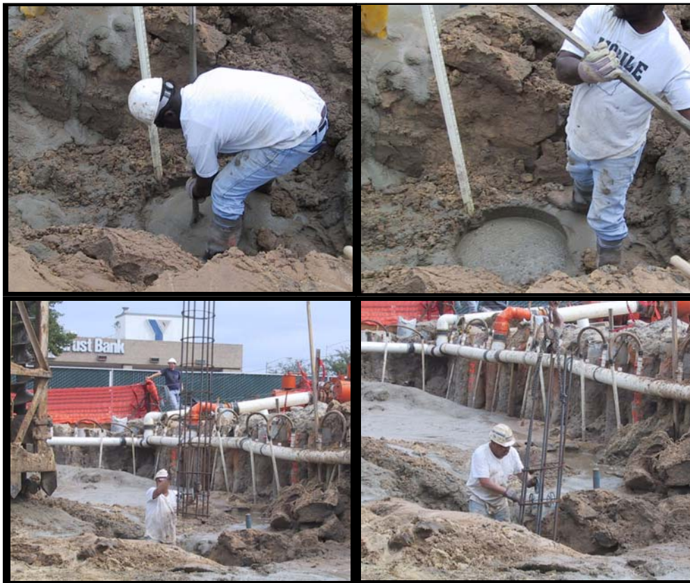
Figure 2.10: Finishing Pile and Reinforcement Placement
