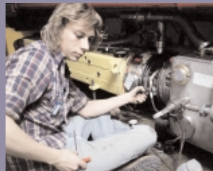
An electrician installs power for the Tevatron.
