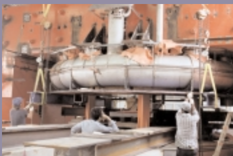
Fixed-target experiment E665 featured the large Chicago cyclotron magnet. The New Muon Building, which houses the magnet to this day, was built around the magnet.
