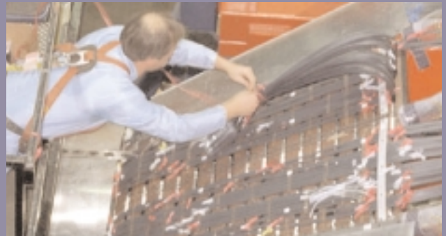
Installing cables in the CDF detector.
