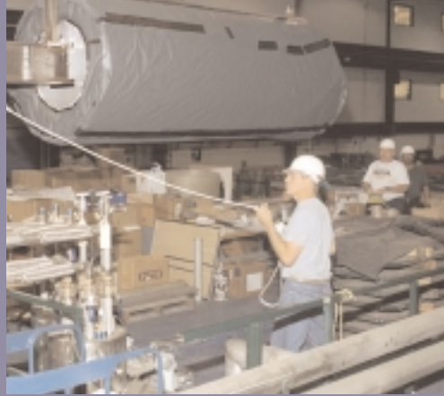
Central Fiber Tracker installation at DZero. Riggers attend to the device as it is moved by crane.
