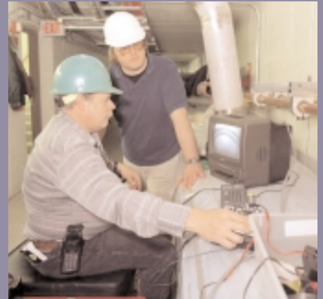
Todd Johnson and Duane Plant examining repairs to Main Injector.
