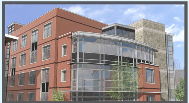
Architects at Bergmann Associates designed Seneca Hall with energy efficiency in mind using EPA's Target Finder. Photo courtesy of Bergmann Associates, SUNY Geneseo, and the Dormitory Authority of the State of New York
