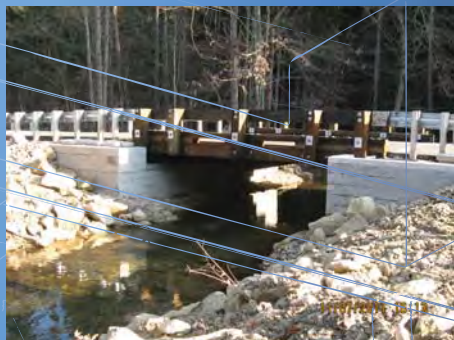
Huston Township, PA GRS Bridge
