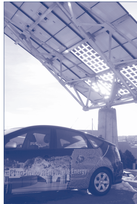
Figure 4: NREL EV/PHEV Charging Tree
