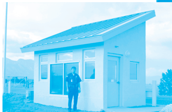
The National Wind Technology Center's site entrance guard post uses passive solar design and roof-integrated solar electricity to significantly reduce utility costs for the building.
