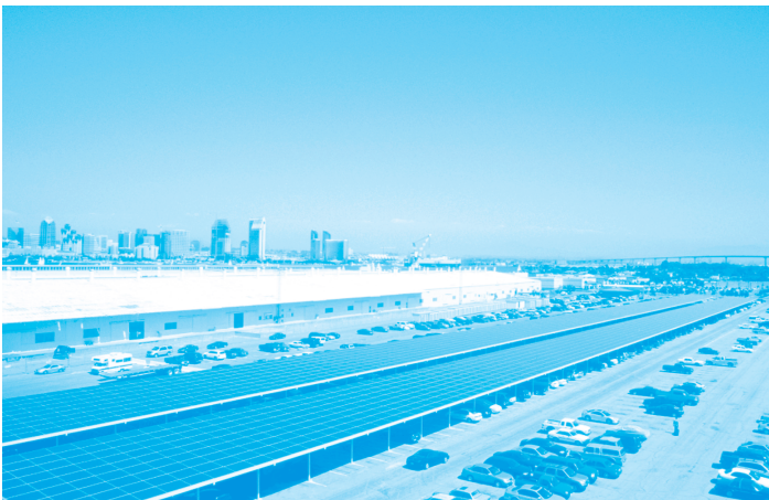
The 750-kilowatt solar electric carport generates power for the Naval Base Coronado while providing more than 400 covered parking spaces for Navy personnel.
