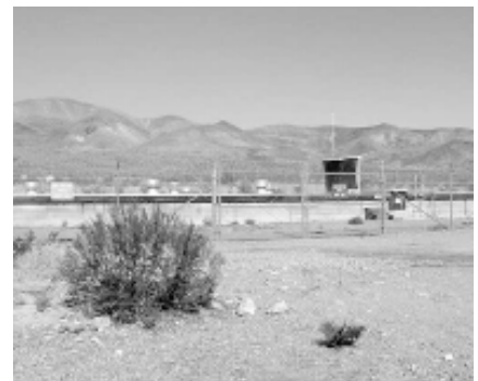
A man-made reservoir at Fort Irwin uses a cooling tower/heat exchanger to help keep the system running smoothly. Water conservation projects at the base are guaranteed to save approximately 121 million gallons of water per year.
