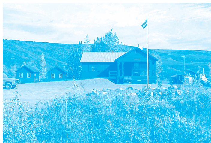
Wonder Lake Ranger Station and outbuildings.
