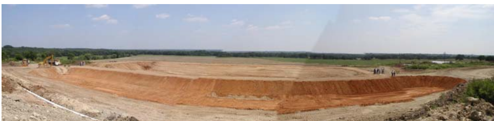
Digester and oxidation pond currently under construction.
