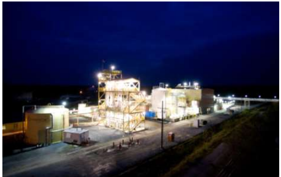
Jennings Demonstration Facility, built and operated by Verenium Corporation
