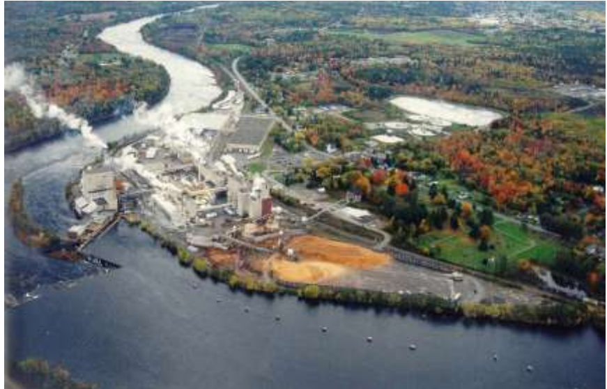
Demonstration of an Integrated Biorefinery at Old Town Maine
