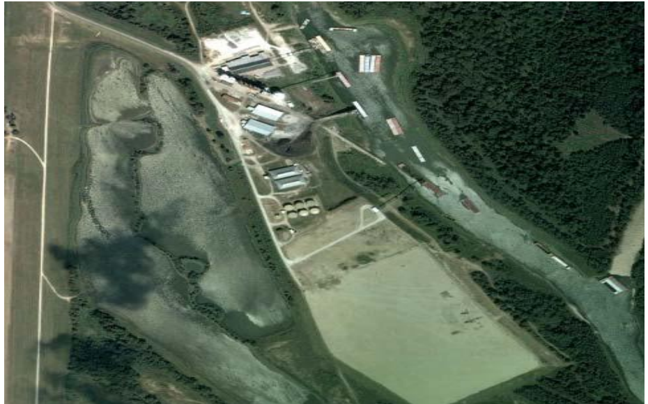
Myriant Succinic Acid Biorefinery Lake Providence, Louisiana site
