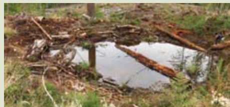
Debris was removed and the depression deepened. Wetland plants were returned, along with some woody debris, and the area was seeded with winter wheat to prevent erosion.
