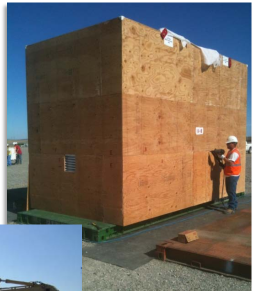
Box Repair at CWC Expansion Area
