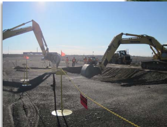
Removing 3 feet Overburden at 3A Trench 8
