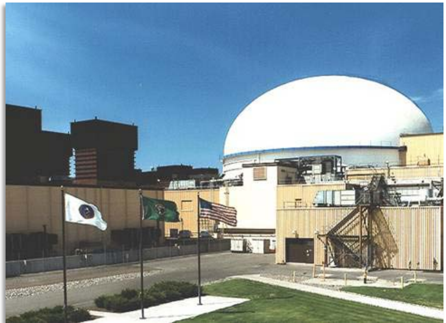
Fast Flux Test Facility
